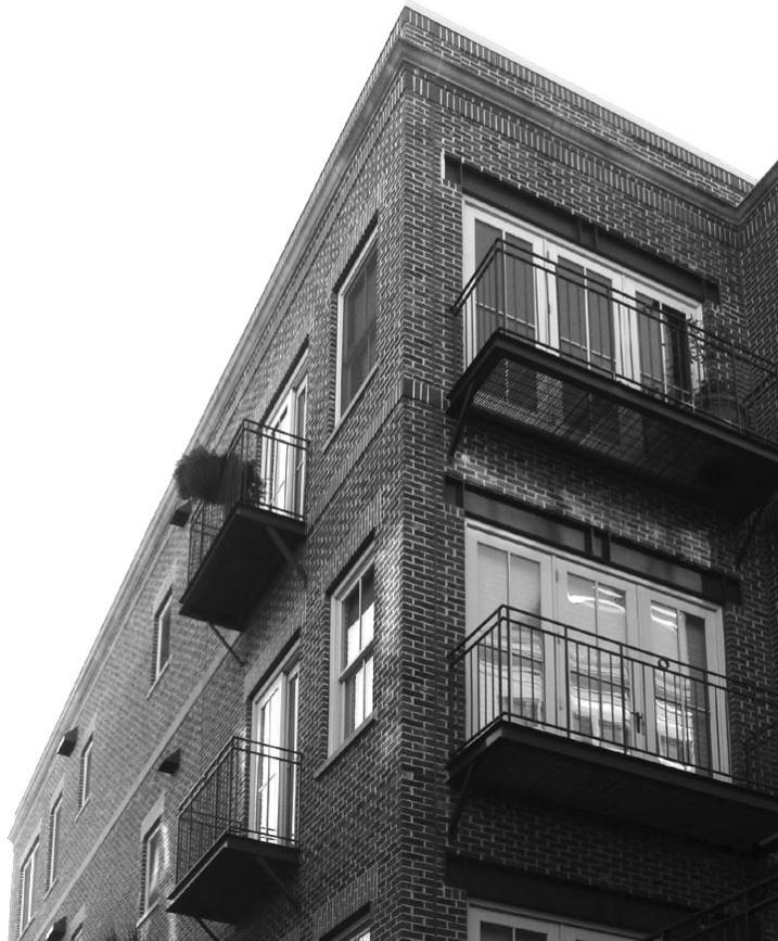
(fig. 4.59) Simple geometric forms and simple plans- waterfront construction, Charleston, SC.
