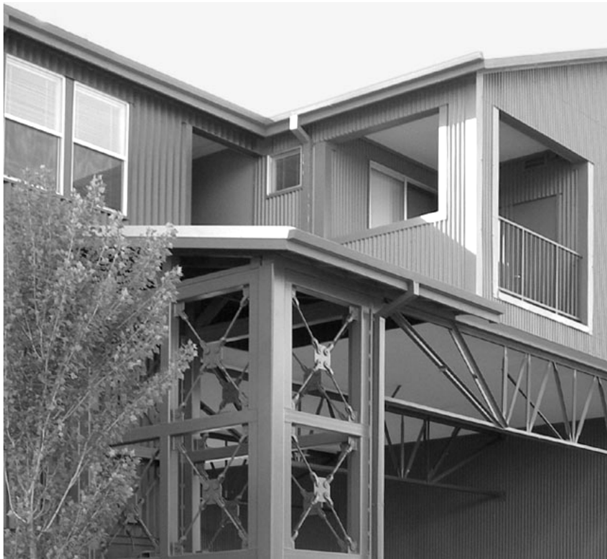
(fig. 4.53) Corrugated metal cladding system used in new construction in warehouse district of Petaluma, CA.
