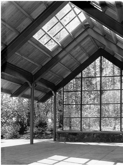
(fig. 4.9) Park pavilion with exposed structural system.
