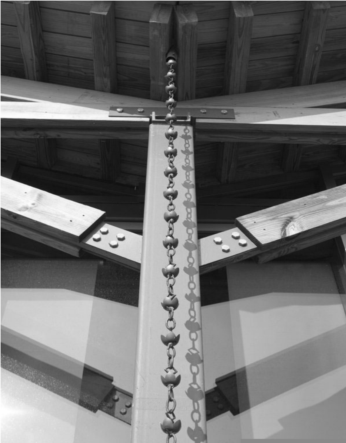
(fig. 4.31) Expression of construction through simple exposed connections (Steel chain rain drip detail - Georgia Environmental Center).
