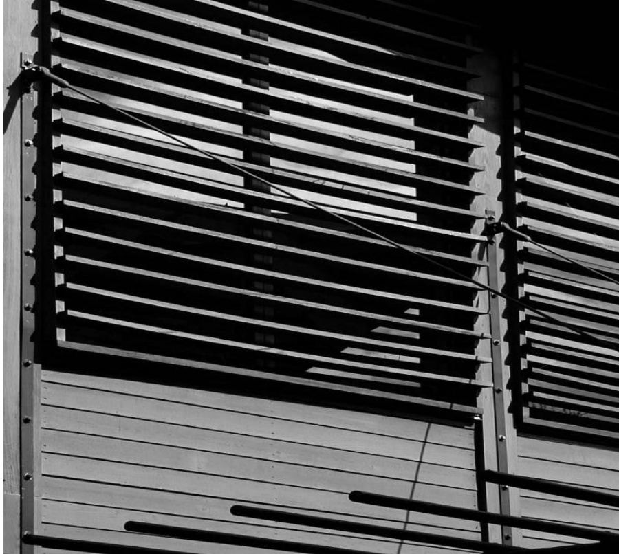
(fig. 4.32) Stained wooden sun screens with steel brackets (Atlantic Center for the Arts, New Smyrna Beach).
