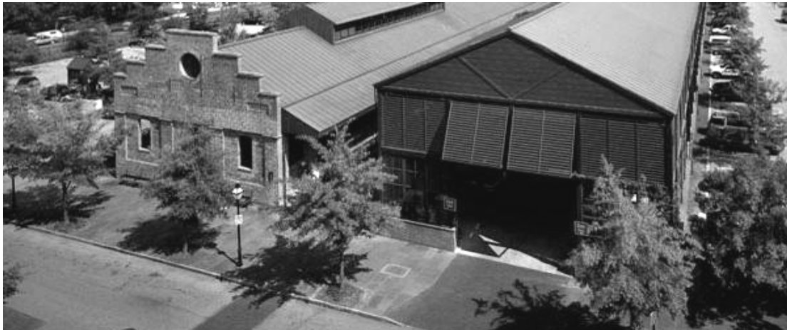
(fig. 4.48) Adapted historic structure (left) and new construction separated by pedestrian corridor in Charleston, SC.
