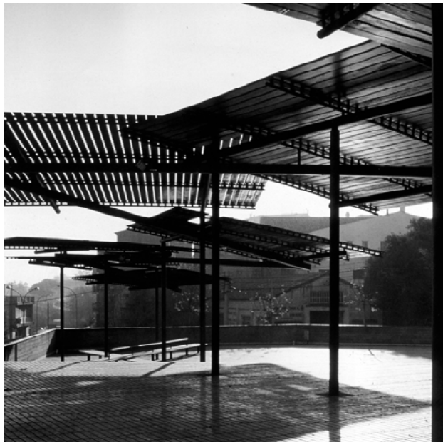
(fig. 4.8) “Artificial trees” in a public space in Spain.
