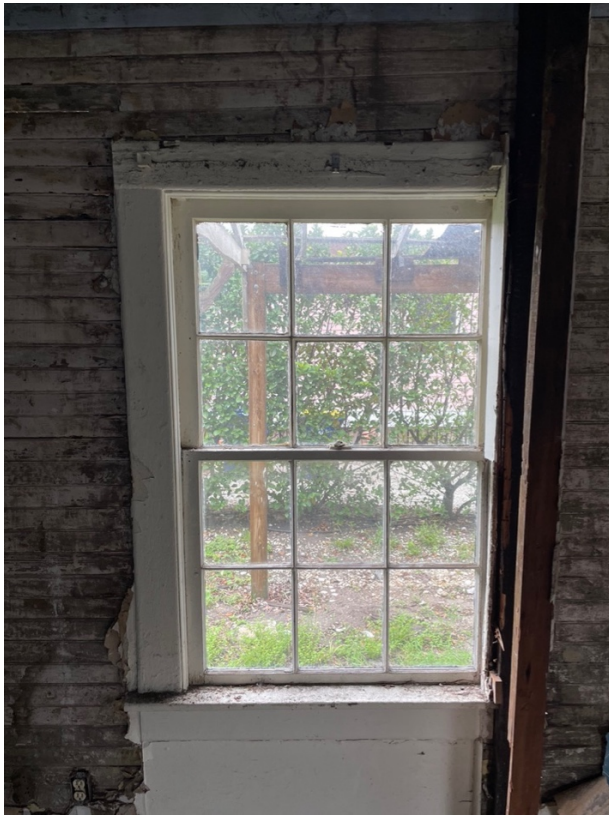
East Elevation: E-2 Interior
