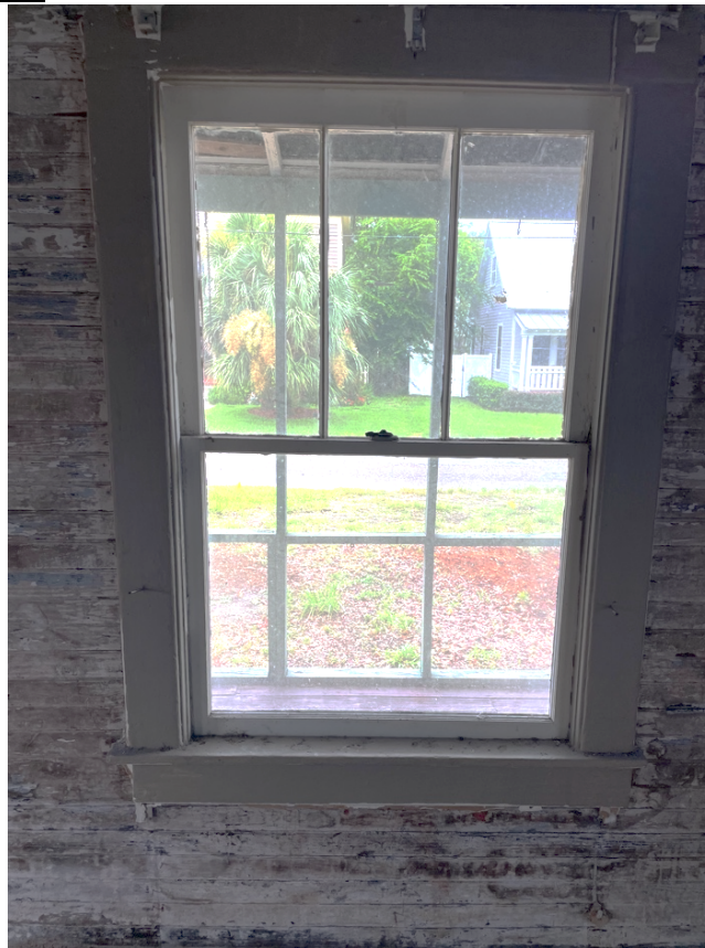
South Elevation Window: S-1 Interior
