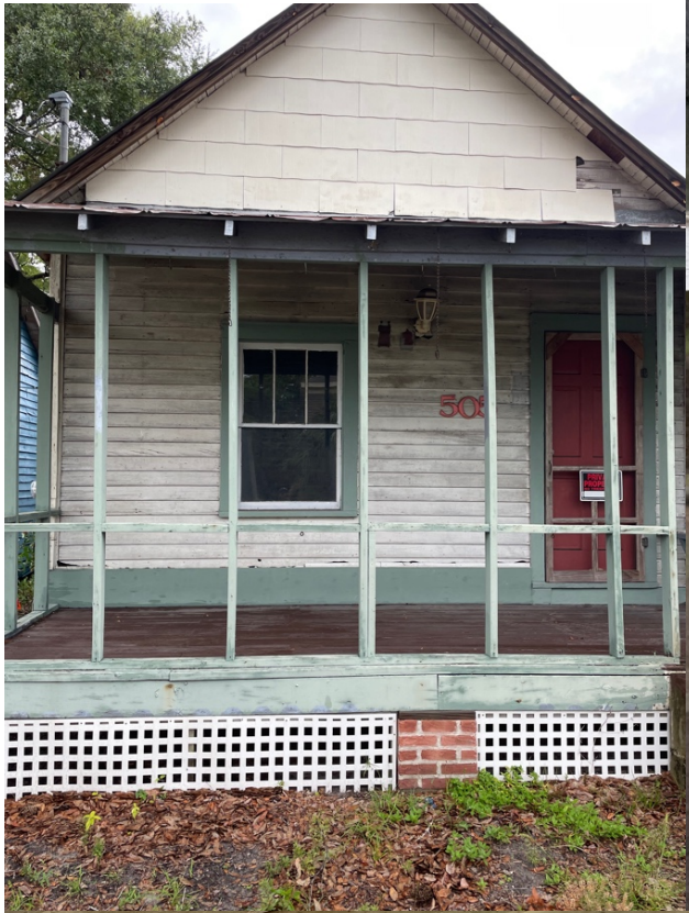
South Elevation Window: S-1 Exterior
