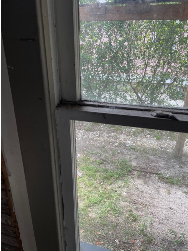
East Elevation: E-1 Interior
