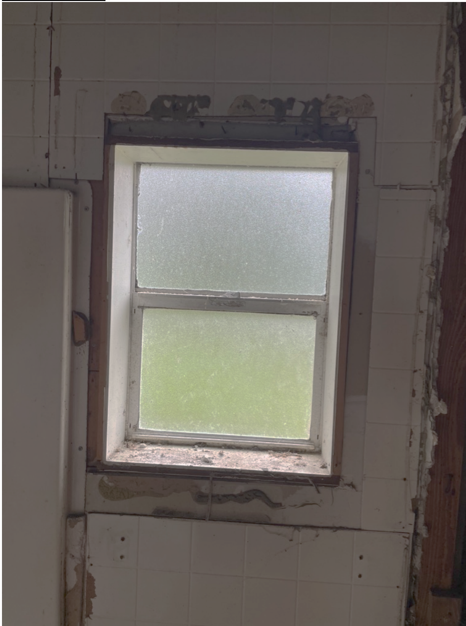
North Elevation: N-1 Interior
