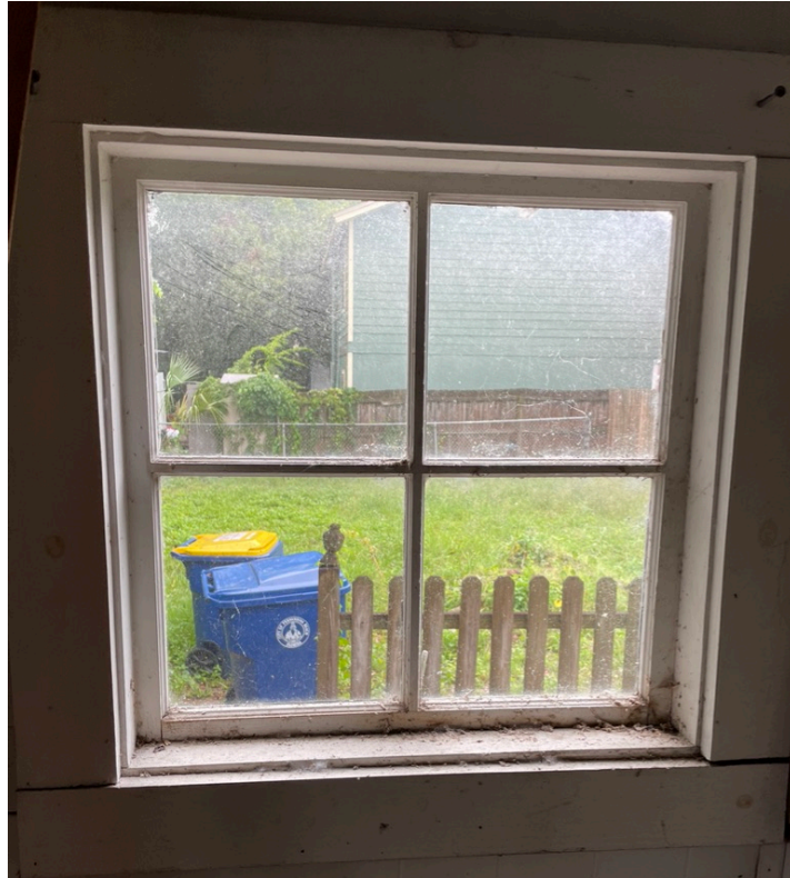
North Elevation: N-2 Interior
