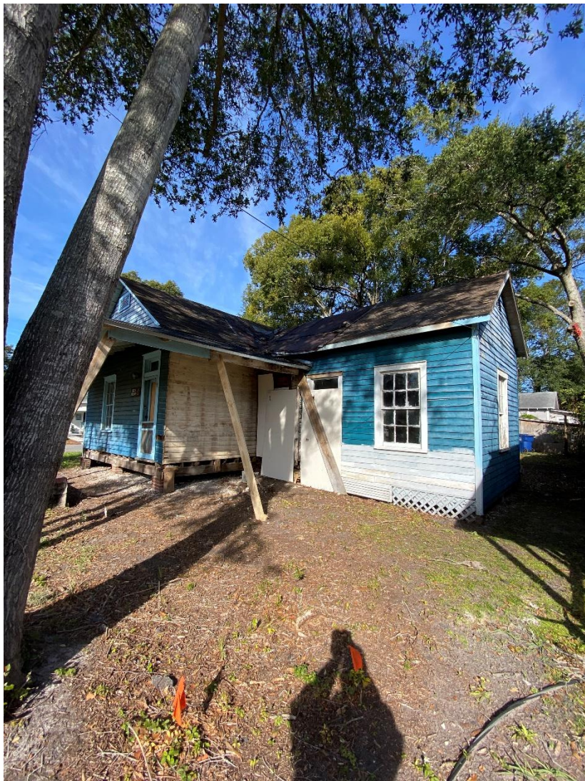
SE Corner – Cedar Street
