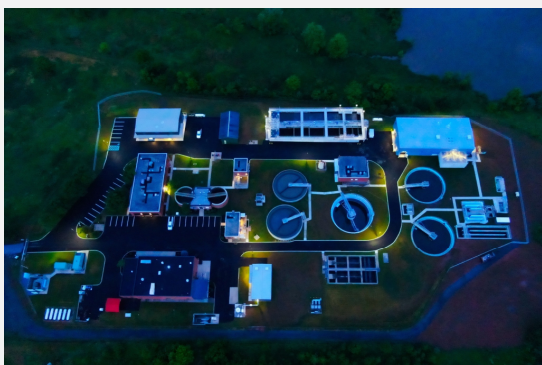
Upper Montgomery Joint Authority, PA WWTP
