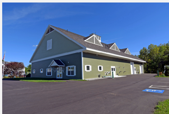
Oxford, ME Membrane Bioreactor WWTF
