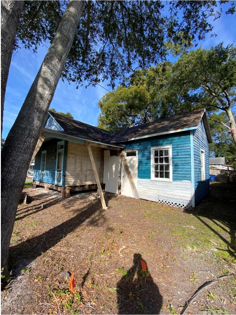
SE Corner – Cedar Street
