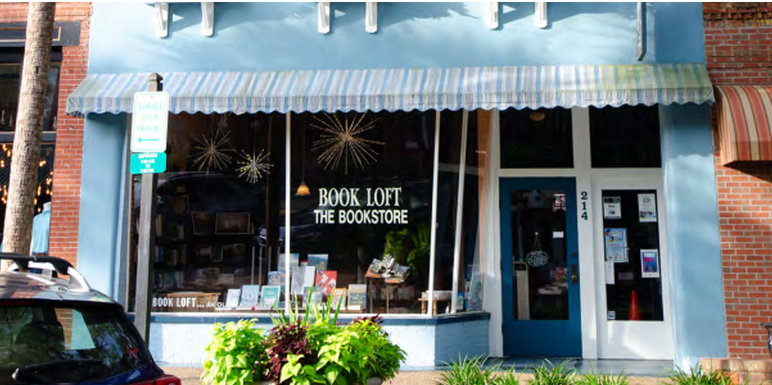
PAINTED EXTERIOR 214 Centre Street
