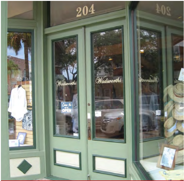
PAINTED EXTERIOR 204 Centre Street
