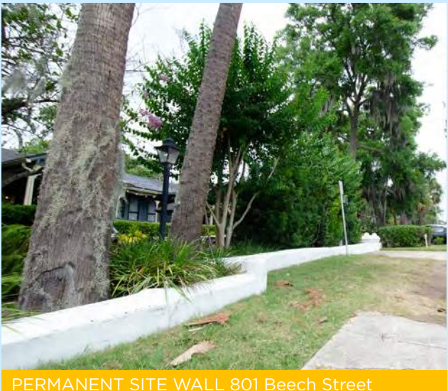
PERMANENT SITE WALL 801 Beech Street
