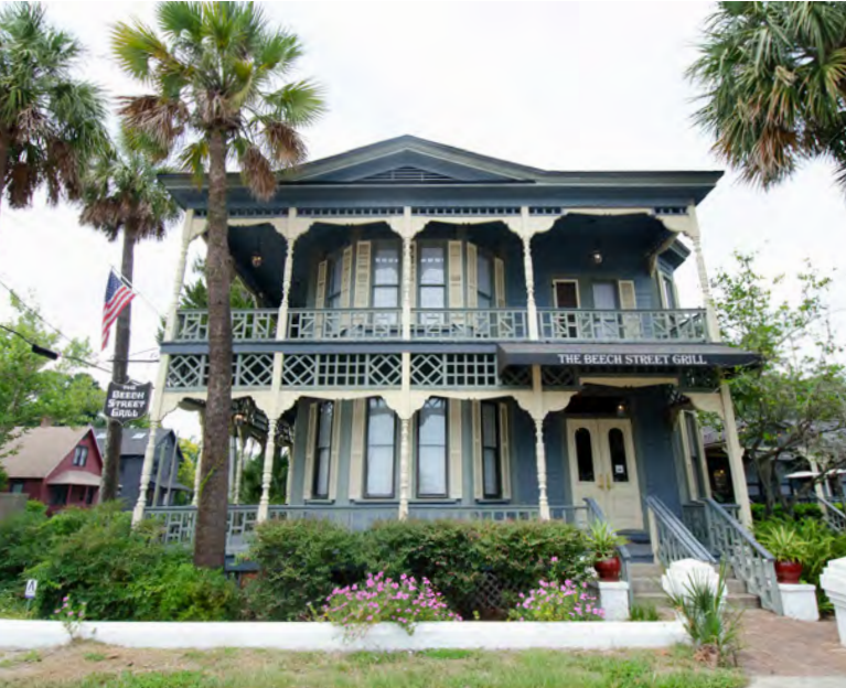
Bell House, 801 Beech Street, 1889: Constructed in 1889 by master builder Captain William Bell, the Bell House is an outstanding example of local millwork. The balustrades on first and second floor porches were inspired by Chinese Chippendale furniture design.
