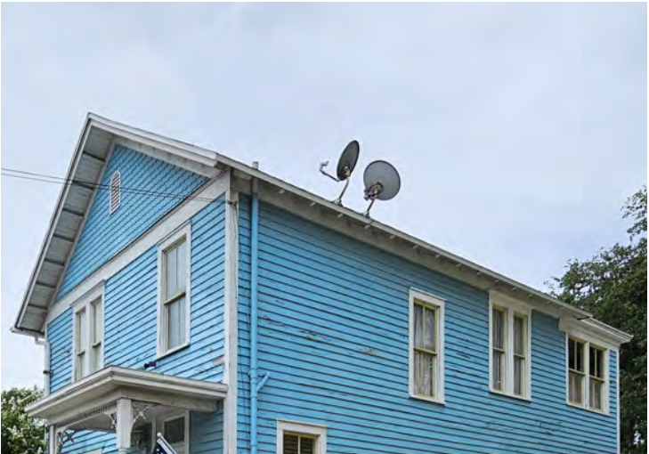
DISH ANTENNAE PLACEMENT 229 South 8th Street
