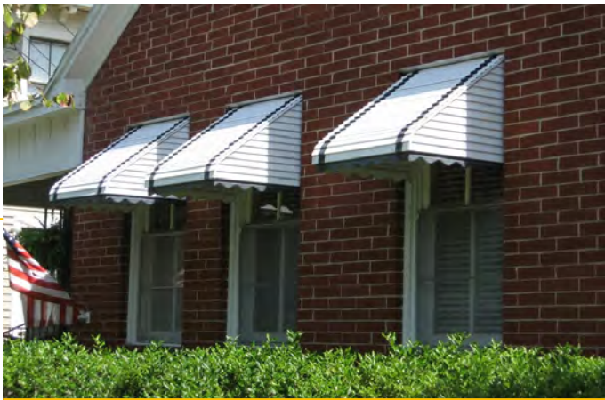
METAL AWNINGS 306 South 7th Street
