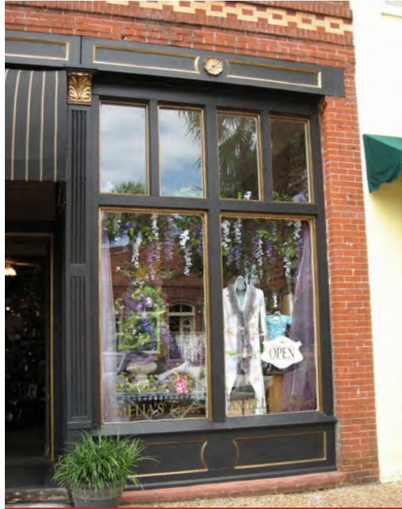
REBUILT STOREFRONT 216 Centre Street
