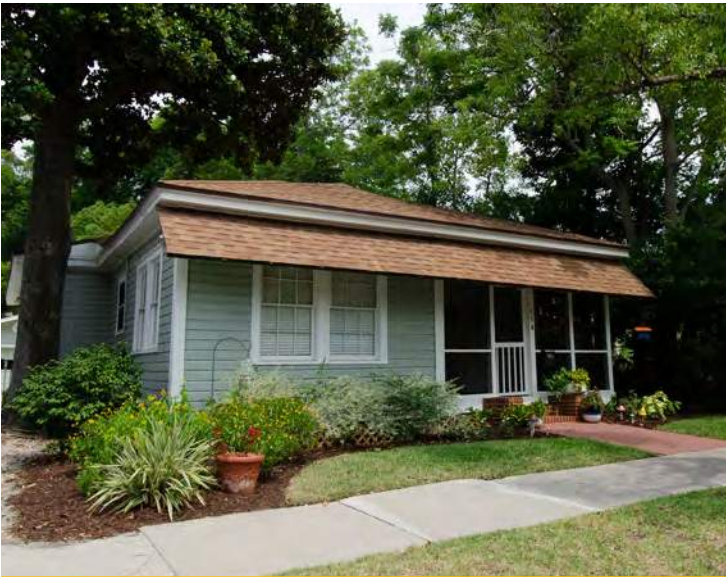
SHED-TYPE AWNING 114 North 3rd Street
