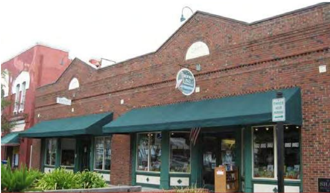
INFILL COMMERCIAL BUILDING 105-107 Centre Street
