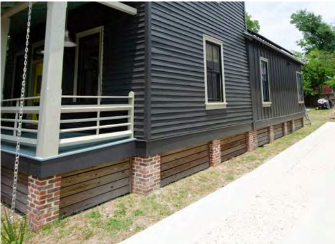
WOOD PANELS 322 North 3rd Street
