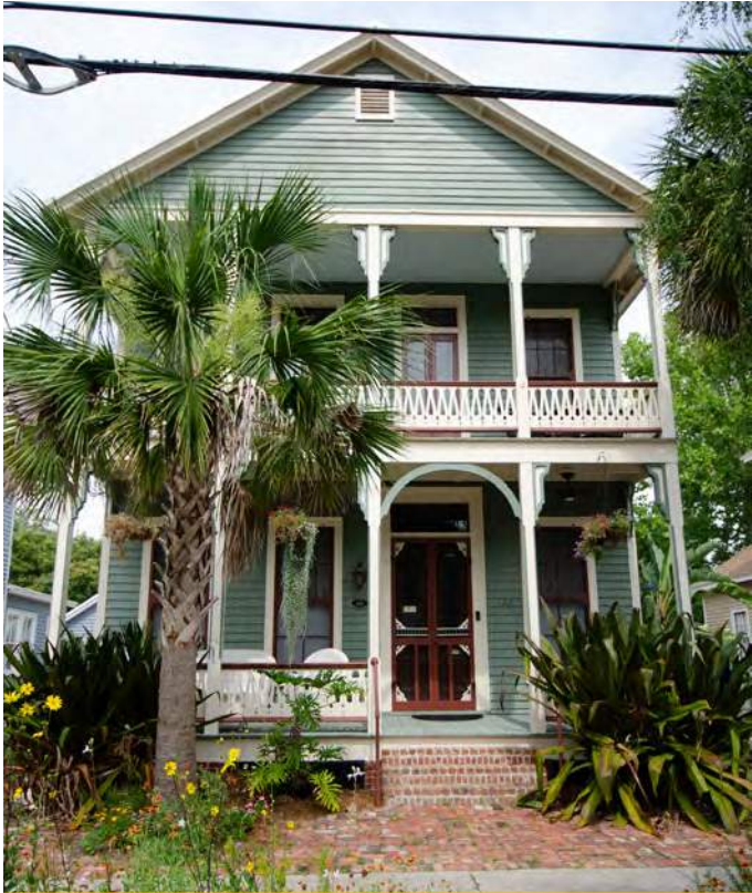
MILLED WOOD PORCH 123 South 7th Street
