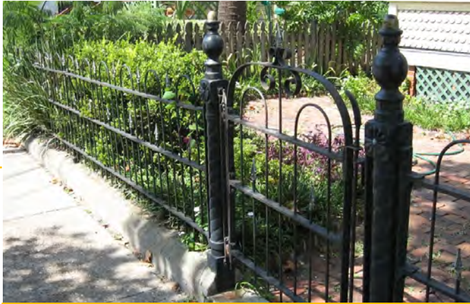
HOOP & DART IRON FENCE 605 Ash Street
