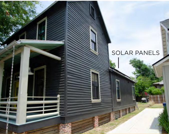
SOLAR PANEL PLACEMENT 322 North 3rd Street
