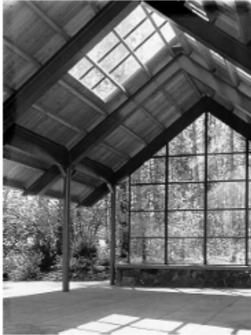
(fig. 4.9) Park pavilion with exposed structural system.
