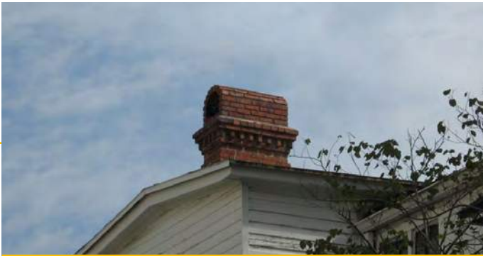
CORBELLED CHIMNEY 415 Centre Street
