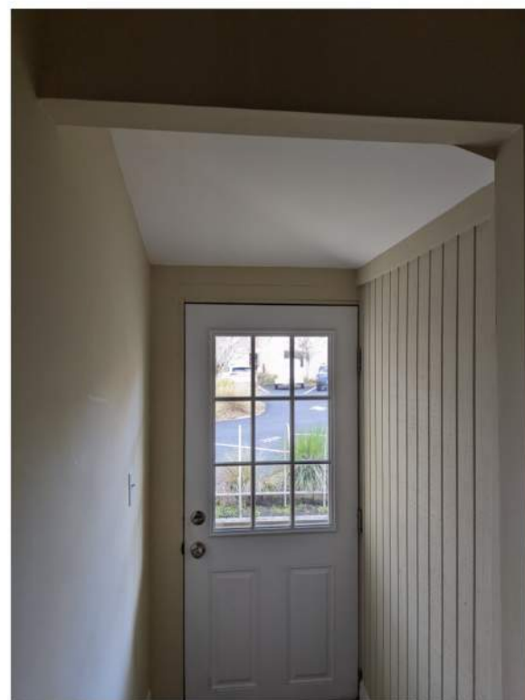
INTERIOR VIEW FROM INSIDE STAIR VIEW OF SHORTENED DOOR HEIGHT TO ACCOMMODATE LOW FRAMED CEILING OFF OF 2X FRAMING.
