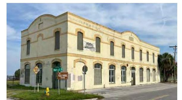
C.H. HUOT BUILDING NOW
