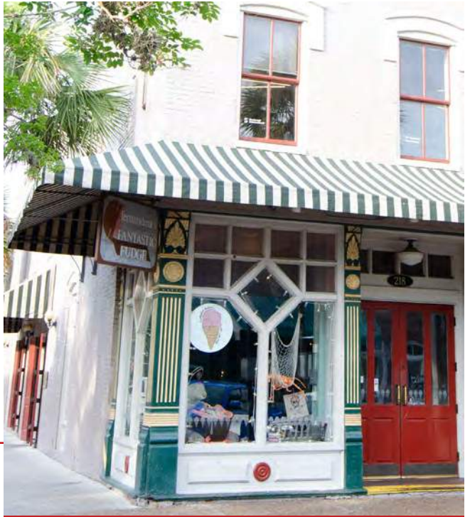
STOREFRONT BULKHEADS 218 Centre Street
