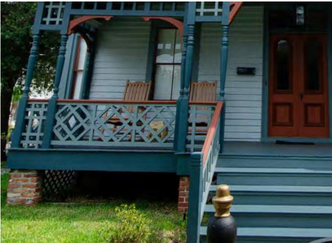
VISIBLE FOUNDATIONS 601 Ash Street
