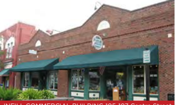
INFILL COMMERCIAL BUILDING 105-107 Centre Street
