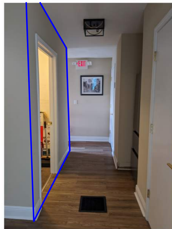
INTERIOR VIEW FROM CORRIDOR THE WALL SHOWN LEFT, PARALLEL TO THE CORRIDOR IS LIKELY NON-BEARING 2X WOOD FRAMED WALL AND WILL BE THE DEMOLISHED AS PART OF THIS NEW WORK.
