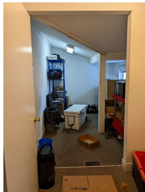
INTERIOR VIEW FROM STORAGE ROOM THIS ALSO HAS A POST COLUMN, NOTE EXTERIOR WALL FINISH AND DIFFERENCE IN FLOOR ELEVATIONS AT THIS LOCATION, MECHANICAL IS FED BELOW ELEVATED FLOOR FRAMING. BEYOND THE DOOR, THIS WALL APPEARS TO BE THE BEARING WALL CONDITION.
