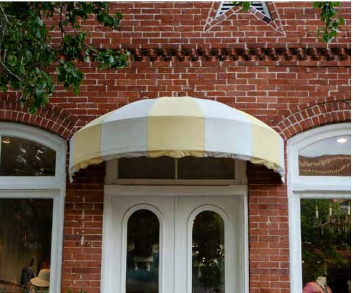
CANVAS SHED AWNING 213 Centre Street
