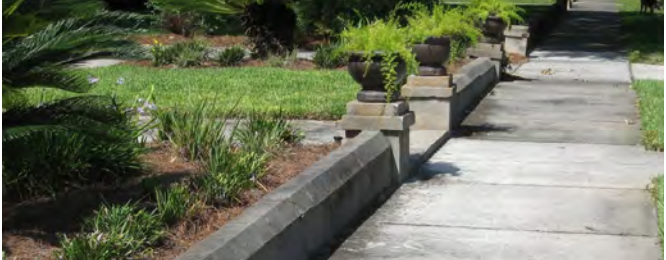
CONCRETE RETAINING WALL 117 North 6th Street
