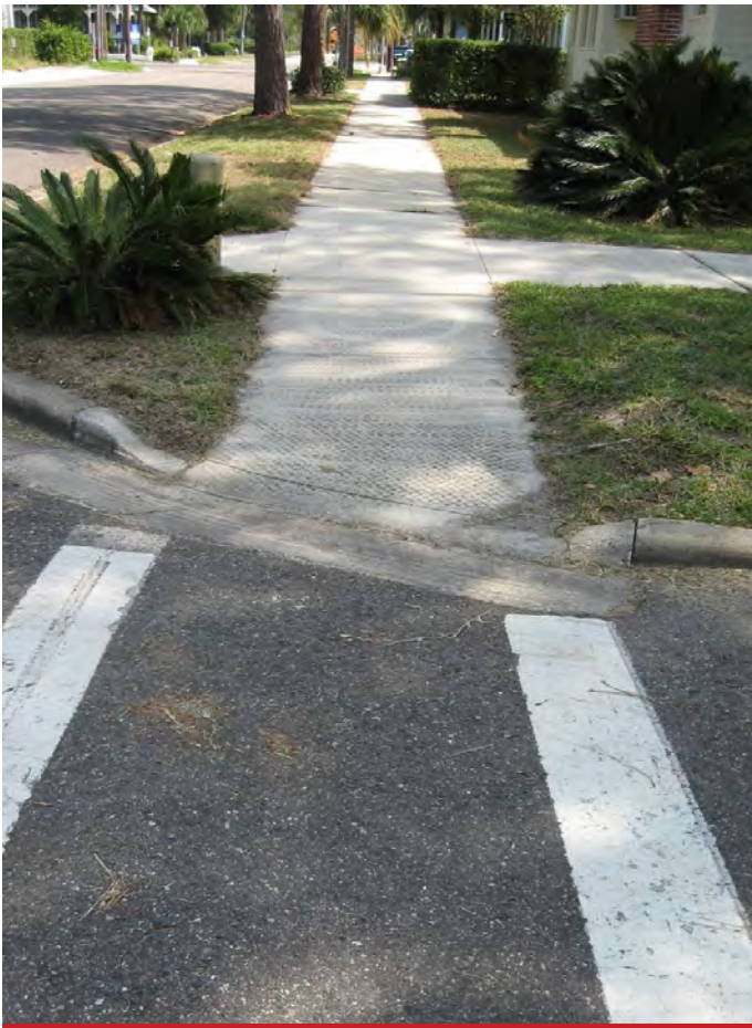
ADA CURBING South 7th Street
