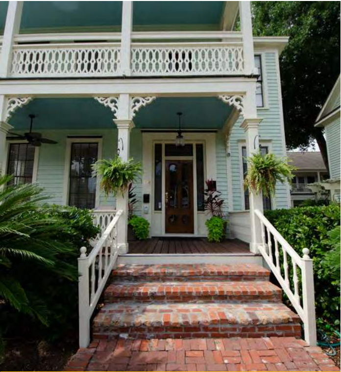
PORCH TRIM 614 Ash Street
