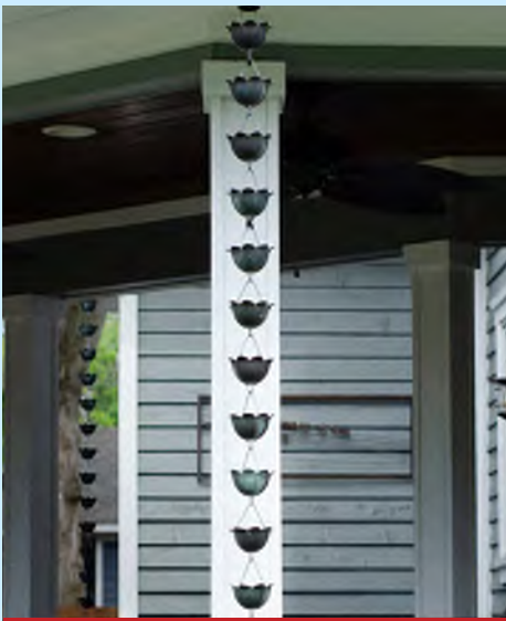
RAIN CHAIN 111 South Seventh Street
