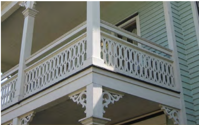
DETAILED WOOD TRIM 121 North 6th Street
