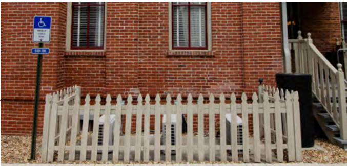
FENCED UTILITIES PLACEMENT EXAMPLE
