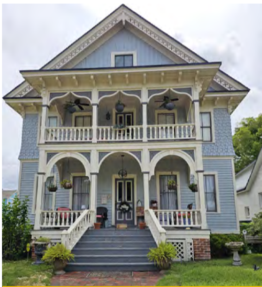
PORCH STAIRS & RAILING 302 South 7th Street
