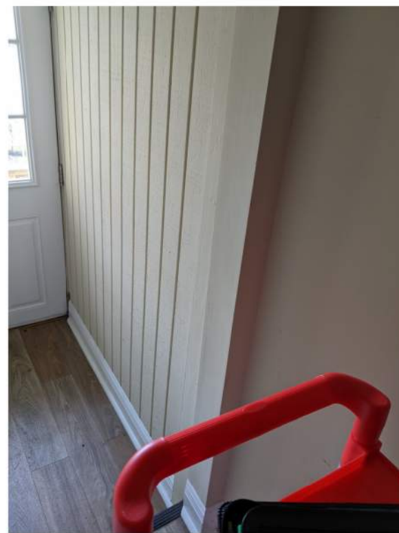
INTERIOR VIEW FROM INSIDE STAIR THERE IS A BUMP IN THE WALL LIKELY A POST COLUMN NOTE EXTERIOR WALL FINISH AND DIFFERENCE IN FLOOR ELEVATIONS AT THIS LOCATION
