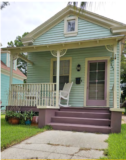
PORCH STAIRS & RAILING 414 South 7th Street
