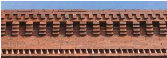
UNPAINTED MASONRY 215-217 Centre St.
