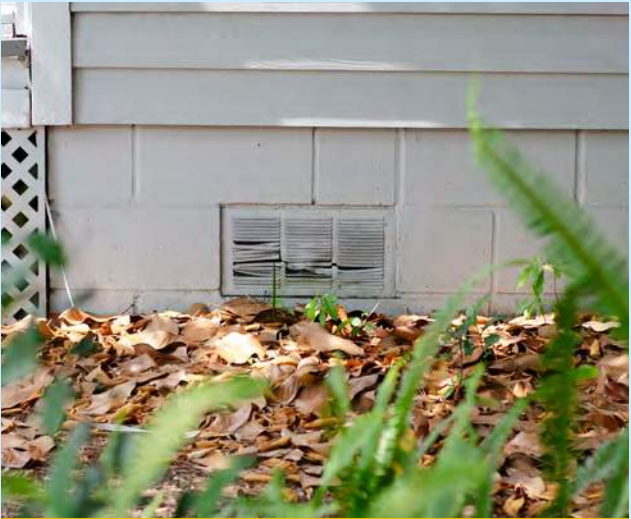
FLOOD VENT 204 South 6th Street
