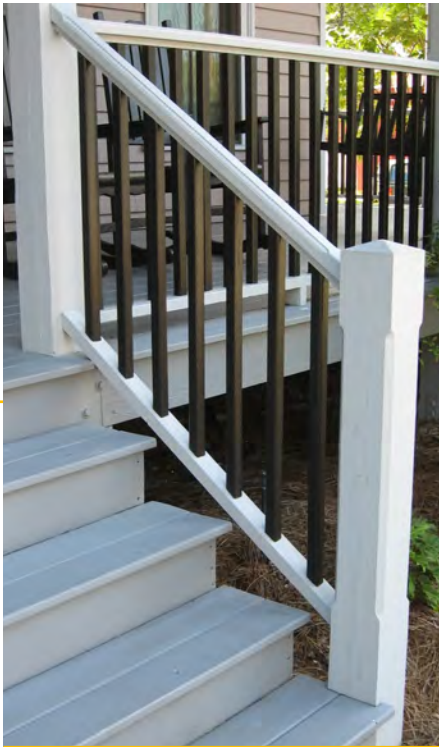
REBUILT PORCH STAIRS & RAILING 604 Ash Street
