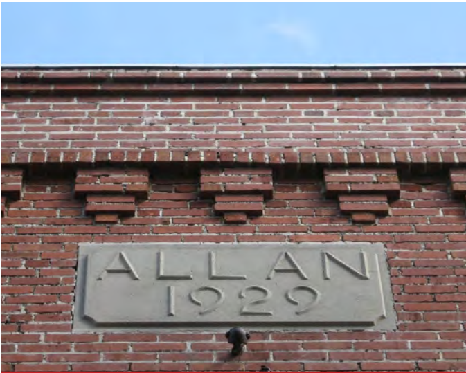
BRICK CORBELLING 309-311 Centre Street
