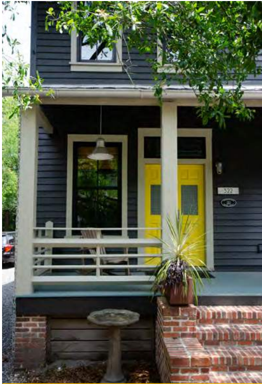
PORCH STAIRS & RAILING 322 N 3rd Street
