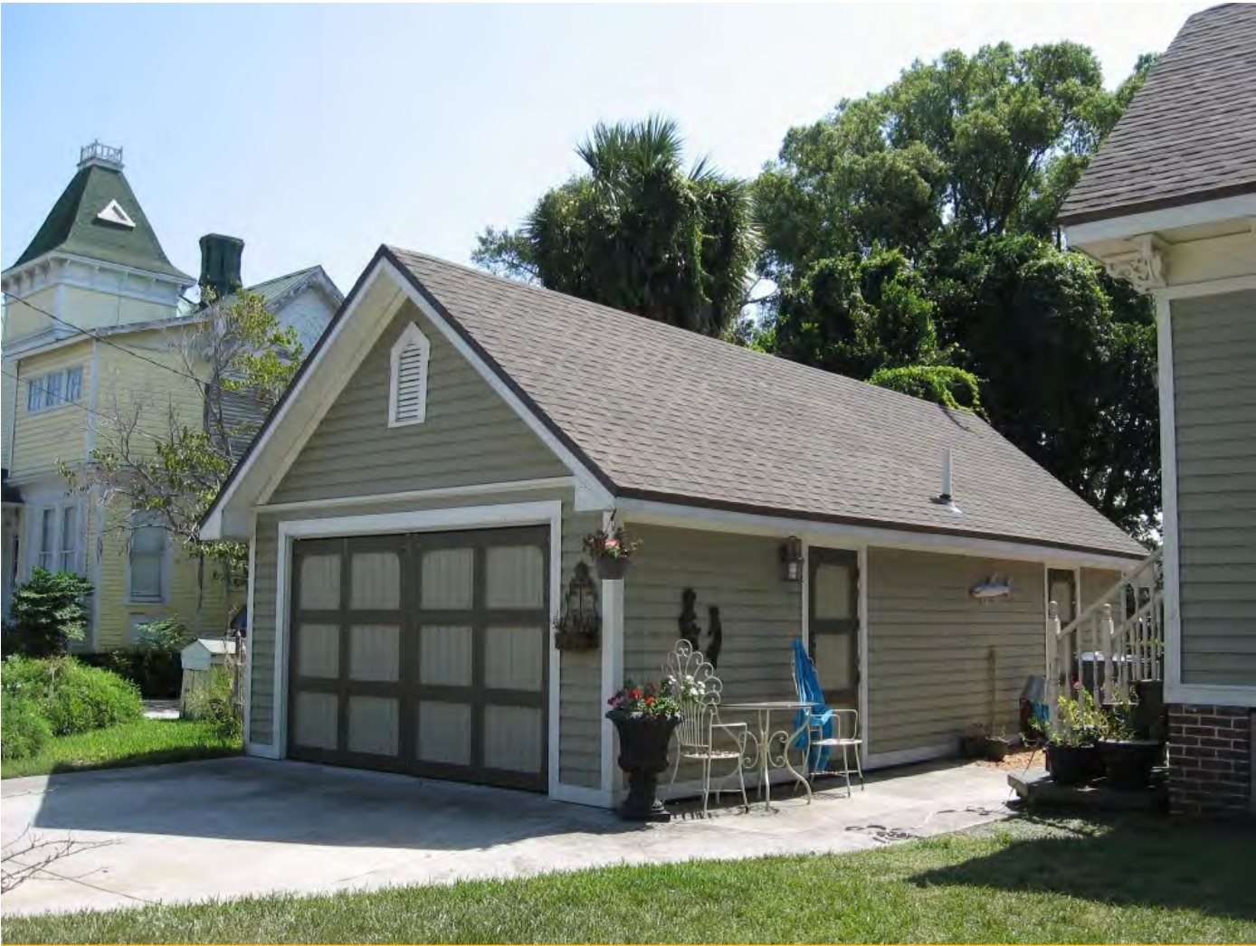
GARAGE OUTBUILDING 302 South 7th Street
