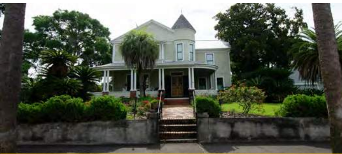
CONCRETE RETAINING WALL 112 North 6th Street
