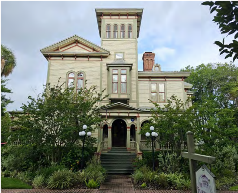
Fairbanks House, 227 S. 7th Street, 1885: Recognized as Florida’s most outstanding example of the Italianate Style, the house know as “Fairbanks Folly,” was designed in 1885 by architect Robert S. Schuyler for George Rainsford Fairbanks. Fairbanks was a pioneer citrus grower, founder and first President of the Florida Historical Society.
