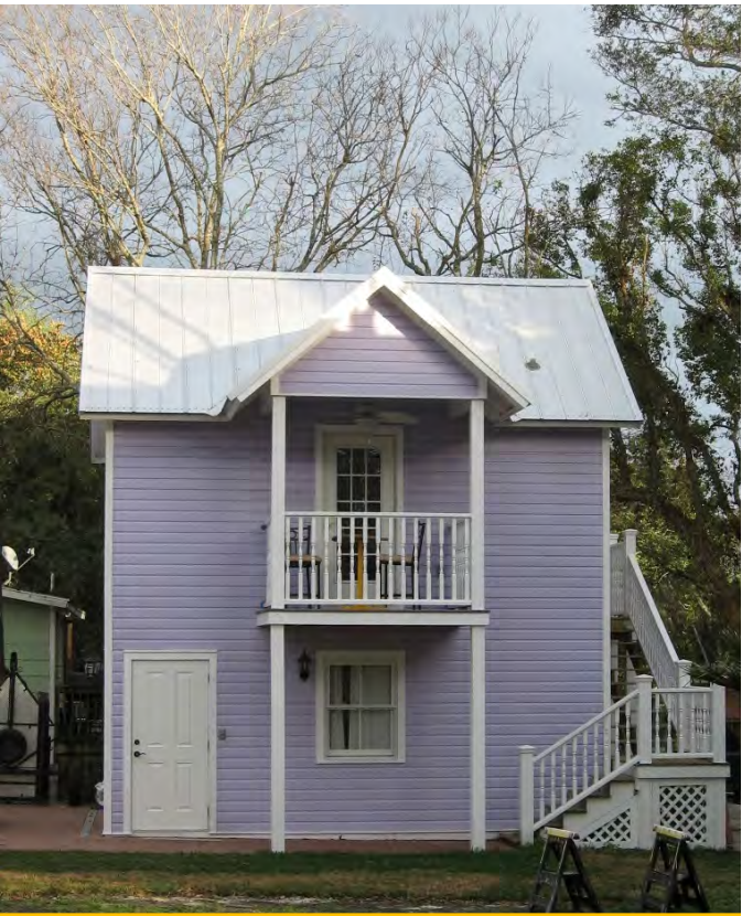
OUTBUILDING DWELLING 432 North 3rd Street
