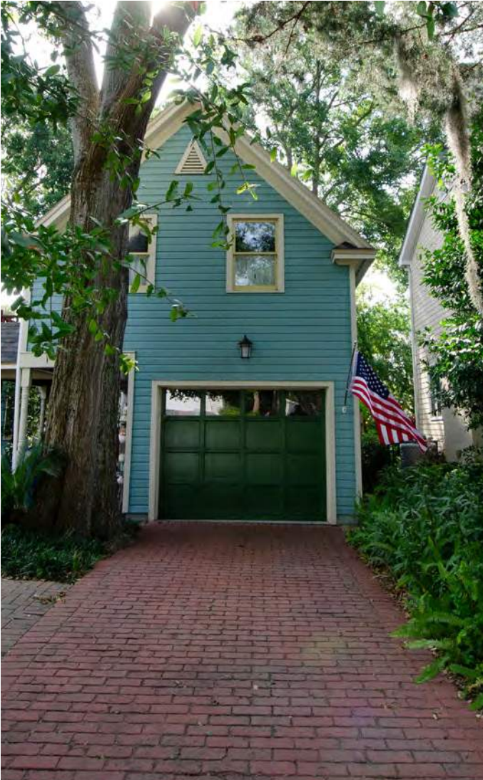
BRICK DRIVEWAY 404 Broome Street
