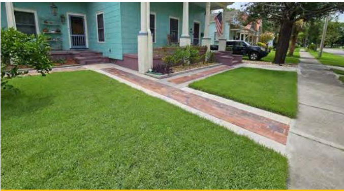
BRICK WALKWAY 410 South 7th Street
