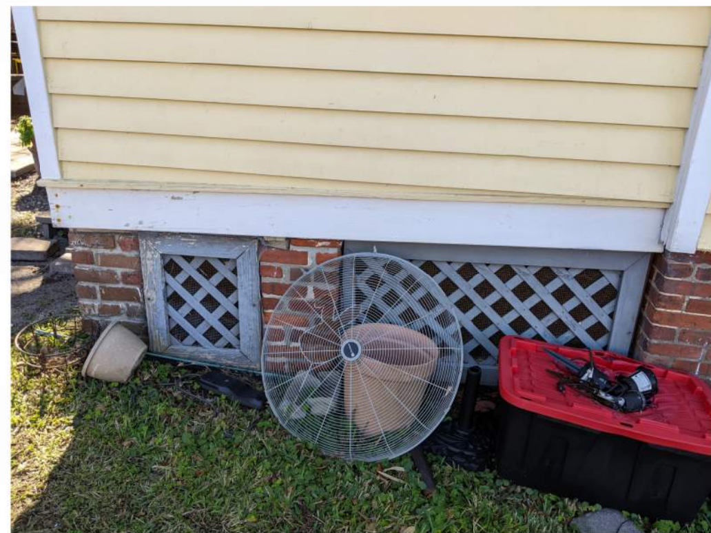
VIEW CLOSEUP OF PILASTERS AND LATTICE SCREEN REFERENCE OF THE SCOPE OF WORK THAT REQUIRES INSPECTION BY A LICENSED ENGINEER PRIOR TO DEMOLITION COMMENCEMENT TO LIMIT RISK TO THE EXISTING STRUCTURE.
