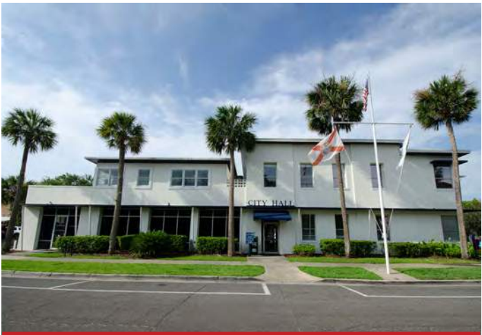
MID CENTURY City Hall, 204 Ash Street
