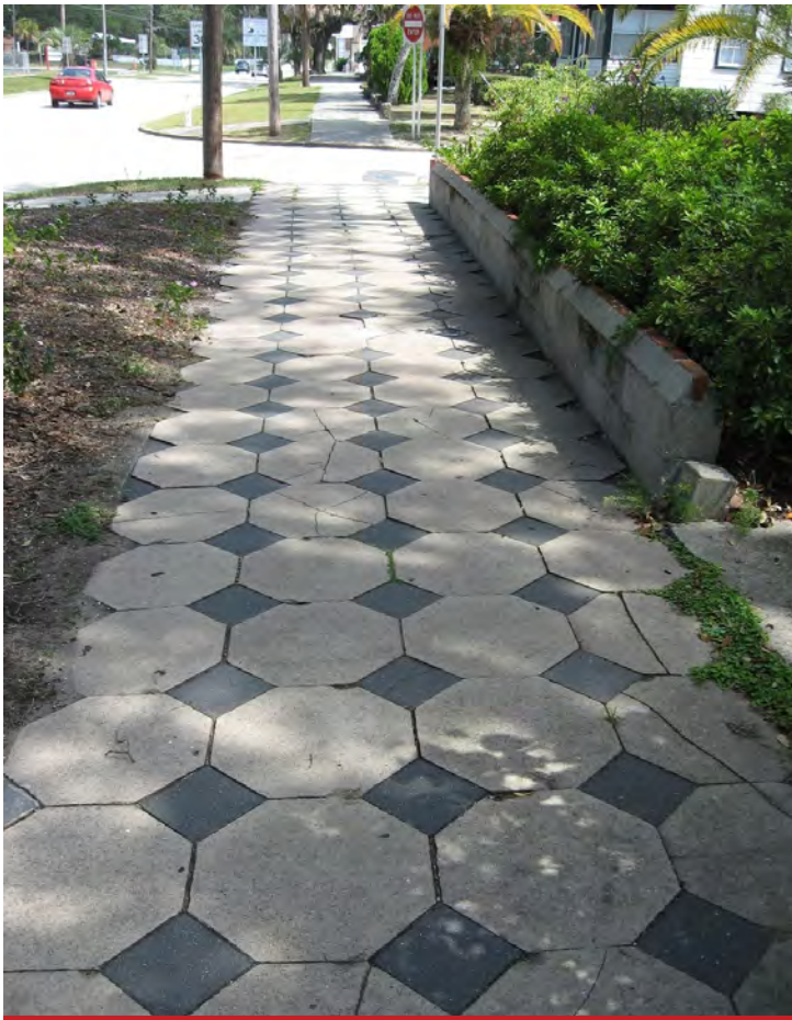
HISTORIC WALKWAY SURFACE 800 Block of Atlantic Ave.
