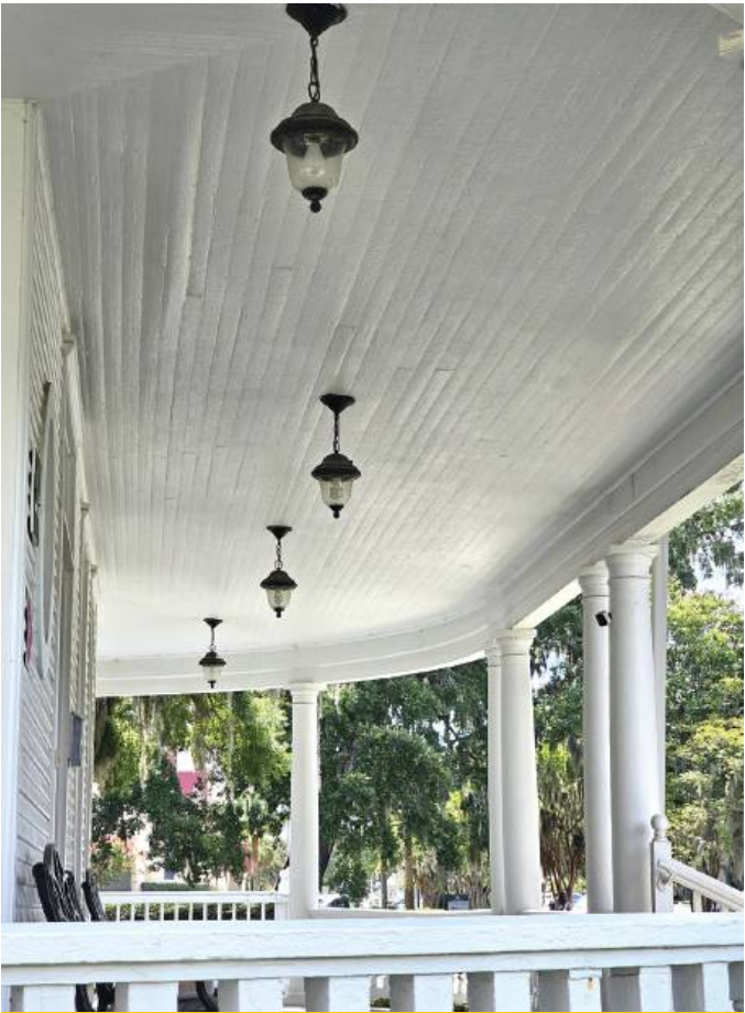
PORCH LIGHT FIXTURE 603 Centre Street
