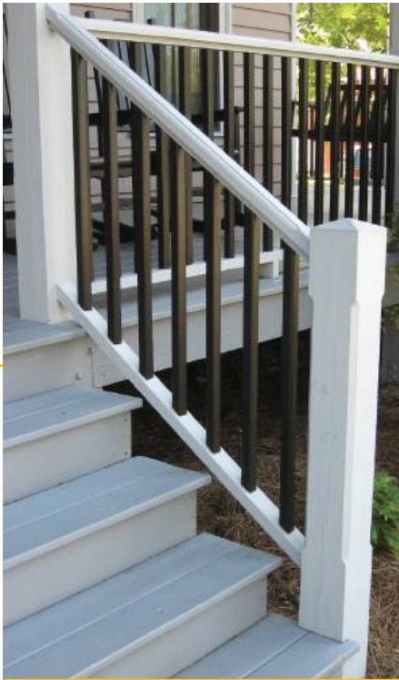
REBUILT PORCH STAIRS & RAILING 604 Ash Street
