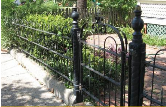
HOOP & DART IRON FENCE 605 Ash Street
