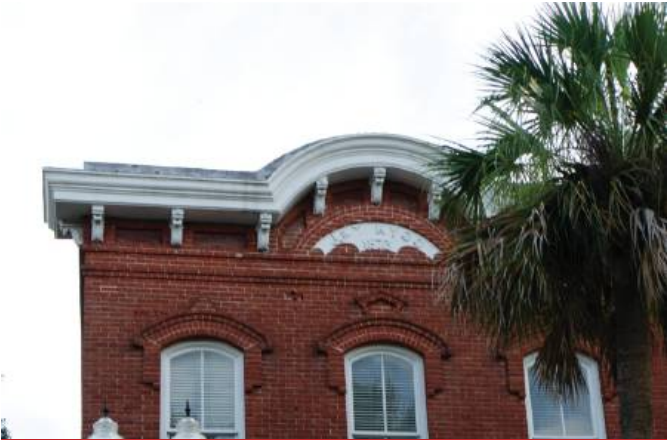
DECORATIVE BRICK CORBELLING 301 Centre Street
