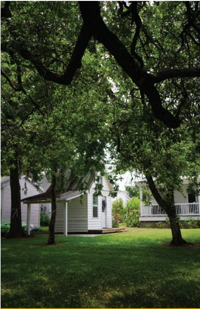
OUTBUILDING SHED 416 North 3rd Street
