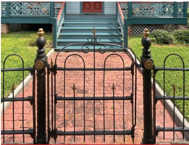
CAST IRON FENCING 601 Ash Street
