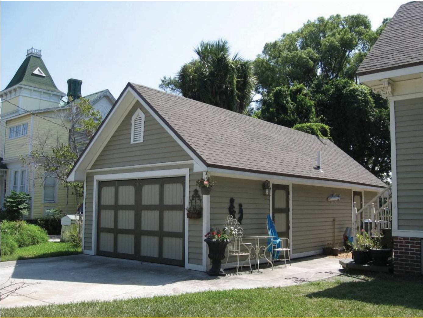
GARAGE OUTBUILDING 302 South 7th Street
