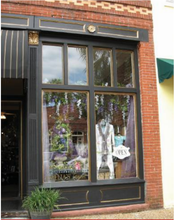
REBUILT STOREFRONT 216 Centre Street
