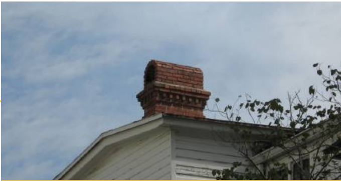
CORBELLED CHIMNEY 415 Centre Street
