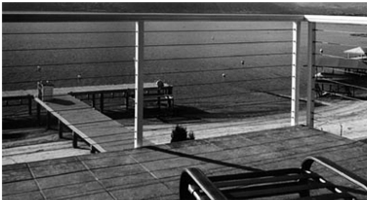
(fig. 4.11) "Cable rail" style railings that provide minimal view interruption and maintains nautical waterfront theme.
