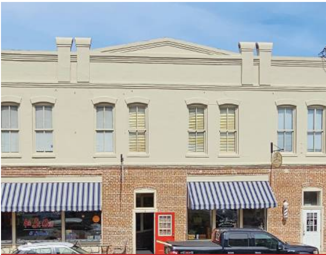
PARAPET & FACADE 3 North 4th Street
