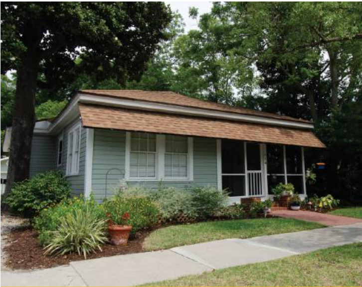
SHED-TYPE AWNING 114 North 3rd Street
