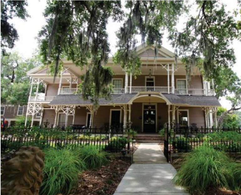
Williams House, 103 S. 9th Street, 1856: One of Fernandina’s oldest buildings, the house was built in 1856 and purchased by Marcellus Williams in 1859. Williams became a wealthy timber baron in partnership with Samuel Swann. Master architect Robert Schuyler designed the wood gingerbread detailing on the porch in the 1880s.
