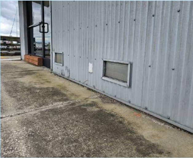
FLOOD VENT 204 South 6th Street
