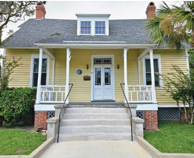
Salvador House, 20 S. 4th Street, c. 1880: Constructed in the early 1880s, by Captain James Bell, a contractor and boat builder, the Salvador House was the home of pioneer Fernandina shrimper Mike Salvador.
