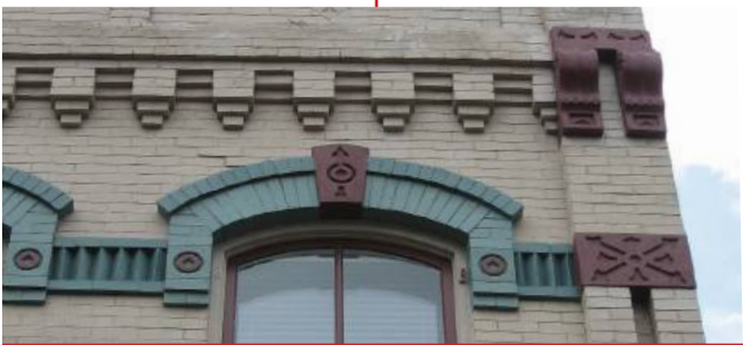
PAINTED BRICK 306 Centre Street
