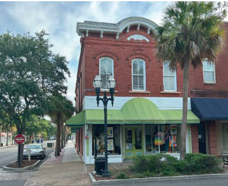
Kydd Building, 301 Centre Street, 1873: The Kydd Building is believed to be the first brick structure on Centre Street. It was constructed in 1873 for James and Thomas Kydd and used as a dry goods store.
