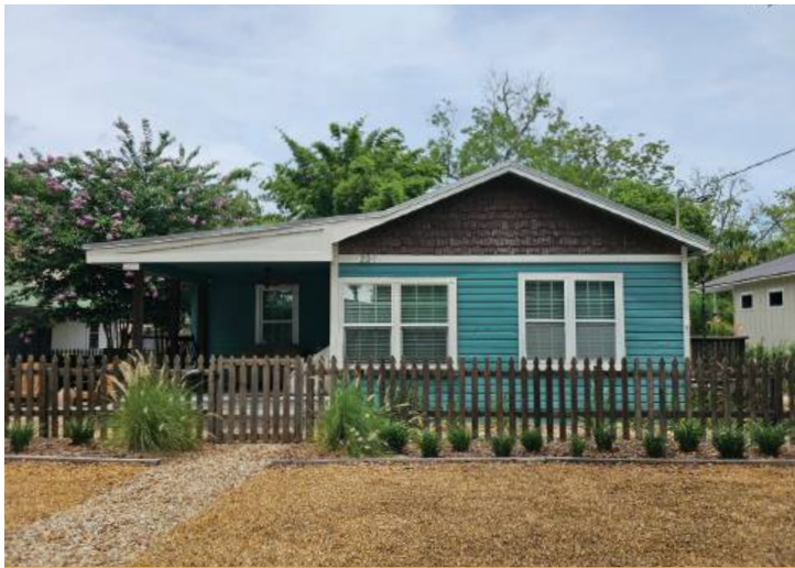
PAINTED WOOD SIDING 221 South 5th Street
