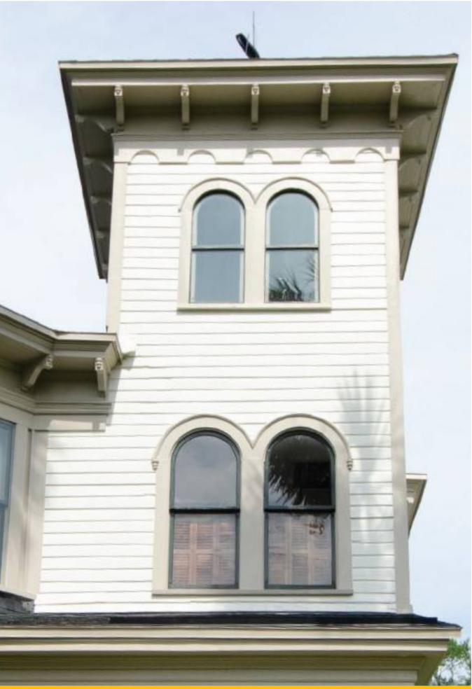
ARCHED WINDOWS 102 North 6th Street
