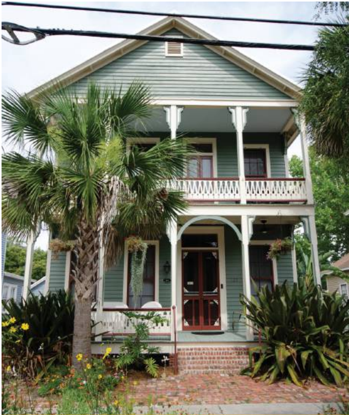
MILLED WOOD PORCH 123 South 7th Street
