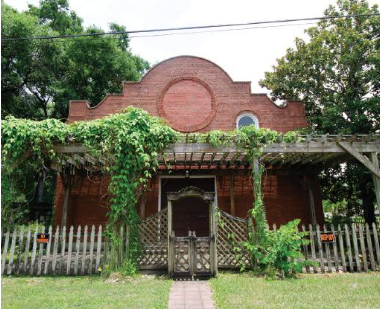
St. Peter's Claver Catholic Church, 302 North 3rd Street, 1910: Built in 1910, this Mission Style building was a highly appropriate design for Fernandina's Black Catholic congregants. Its main façade features a character defining curvilinear parapet and arched windows.
