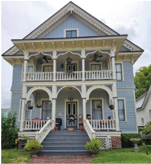
PORCH STAIRS & RAILING 302 South 7th Street
