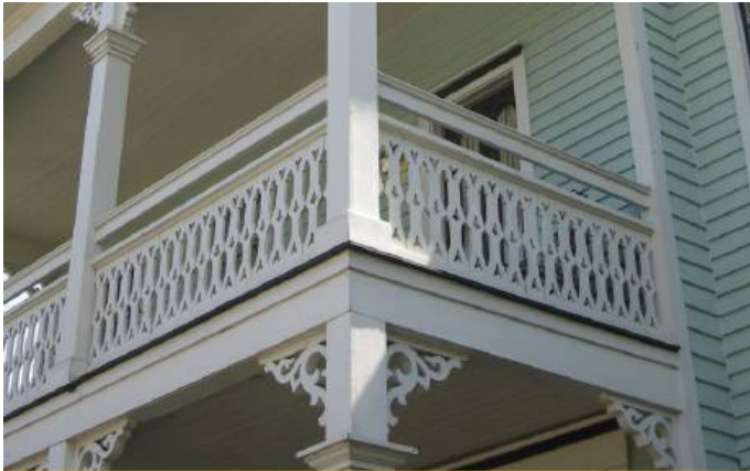
DETAILED WOOD TRIM 121 North 6th Street
