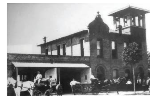
CITY HALL STRUCTURE IN 1915
