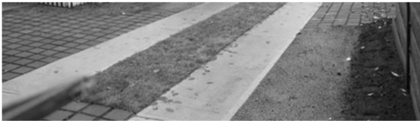
(fig. 5.12) Pervious parking surfaces.
