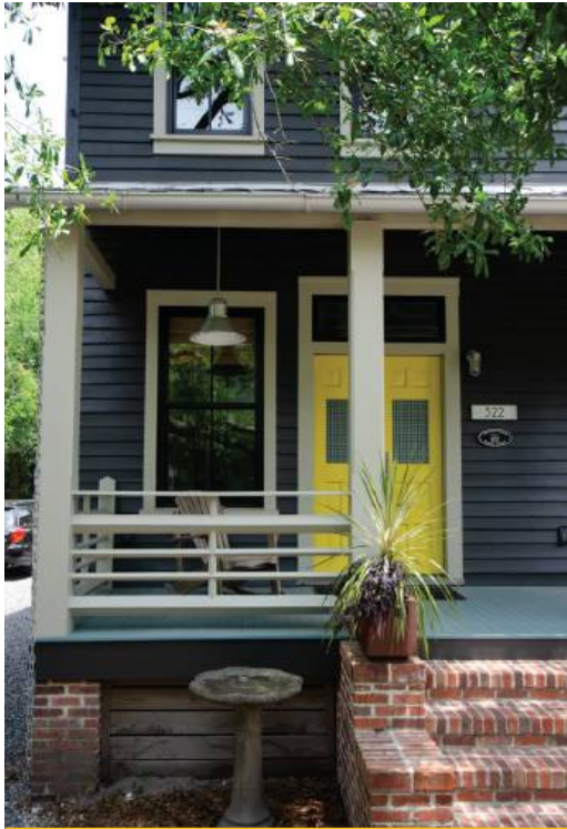
PORCH STAIRS & RAILING 322 N 3rd Street
