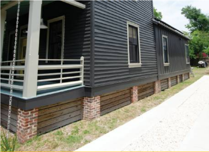
WOOD PANELS 322 North 3rd Street
