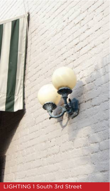
LIGHTING 1 South 3rd Street Early 20th Century
