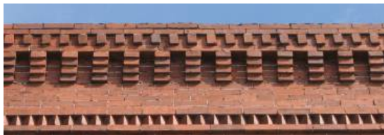
UNPAINTED MASONRY 215-217 Centre St.
