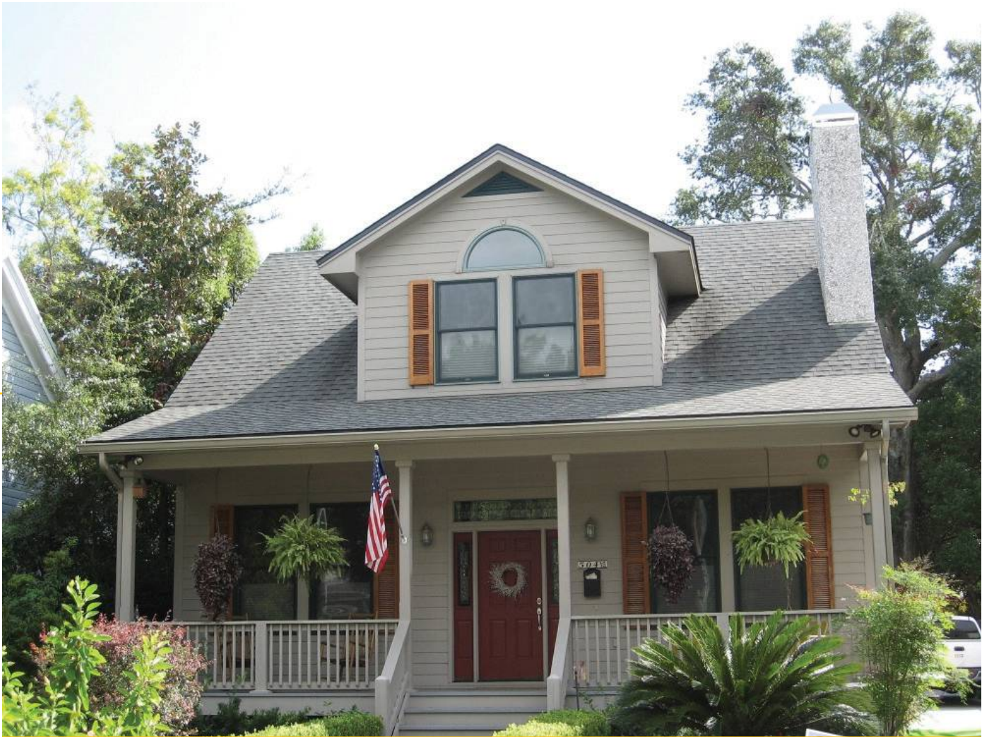
RECENTLY BUILT DWELLING EXAMPLE 504 Beech Street
