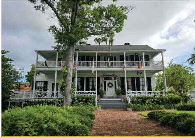
BRICK WALKWAY 415 Centre Street
