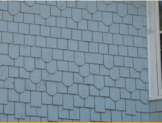
WOODEN SHINGLES 214 South 7th Street
