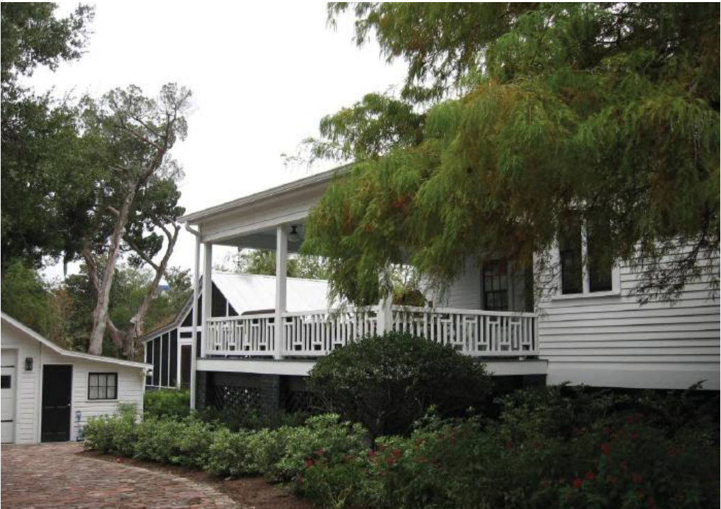
REAR PORCH ADDITION 120 North 6th Street
