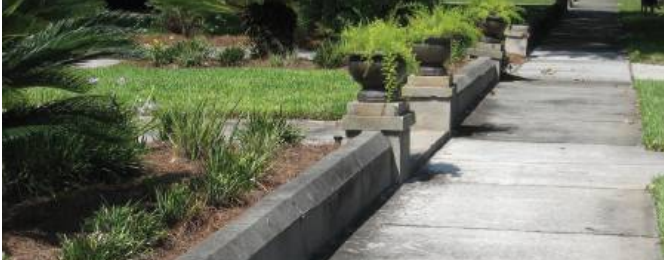
CONCRETE RETAINING WALL 117 North 6th Street
