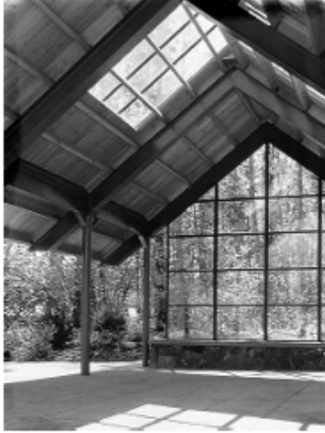
(fig. 4.9) Park pavilion with exposed structural system.
