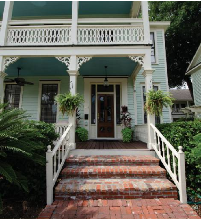
PORCH TRIM 614 Ash Street
