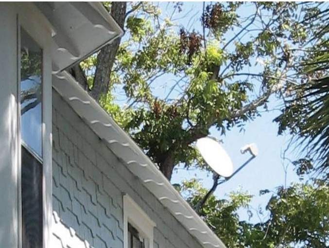
DISH ANTENNAE PLACEMENT 214 South 7th Street
