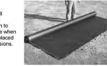
Figure 4.3d. Stabilized Construction Exit
