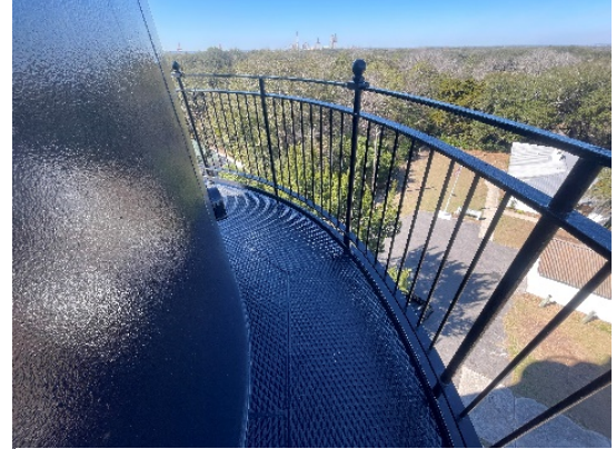
Photo 17 (Left): View of cast iron elements crowning the historic lighthouse structure. Minor, isolated corrosion stains were observed at the top, near cast iron structural supports.
