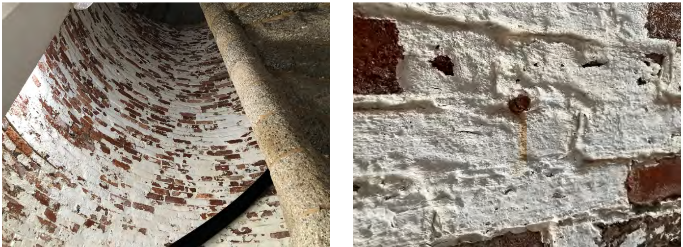
Photo 7: Interior view of painted brick masonry surfaces, looking up the lighthouse staircase.
