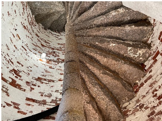
Photo 1: Interior of Amelia Lighthouse, with granite stair treads and painted brick masonry.
