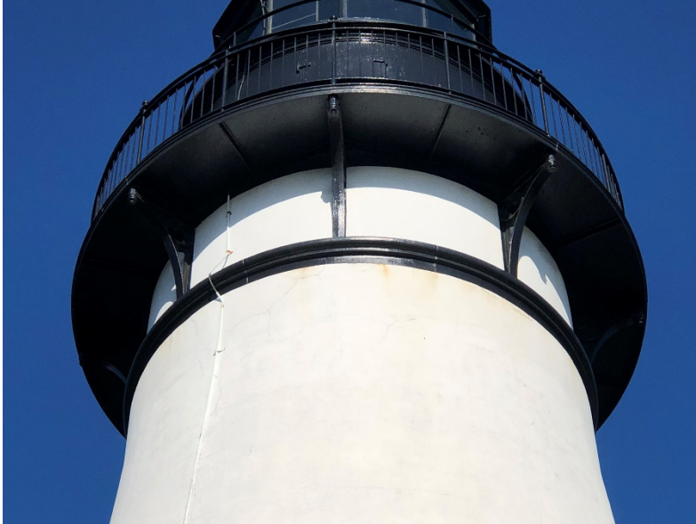
Photo 17 (Left): View of cast iron elements crowning the historic lighthouse structure. Minor, isolated corrosion stains were observed at the top, near cast iron structural supports.
