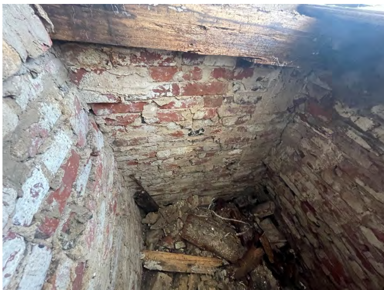
Photo 20: View, from interior, of exterior wall (at right) and interior wall (at left), connected by perpendicular brick masonry wall (at center).
