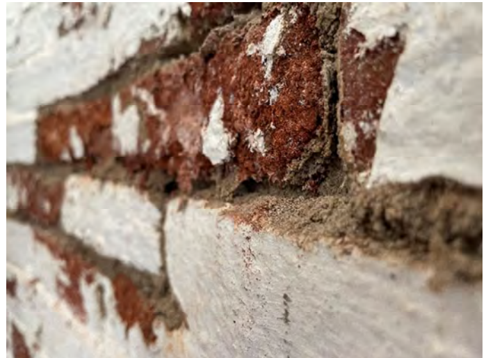
Photo 3: Typical condition of an original lime mortar joint, with some mortar erosion visible, observed at interior wall.
