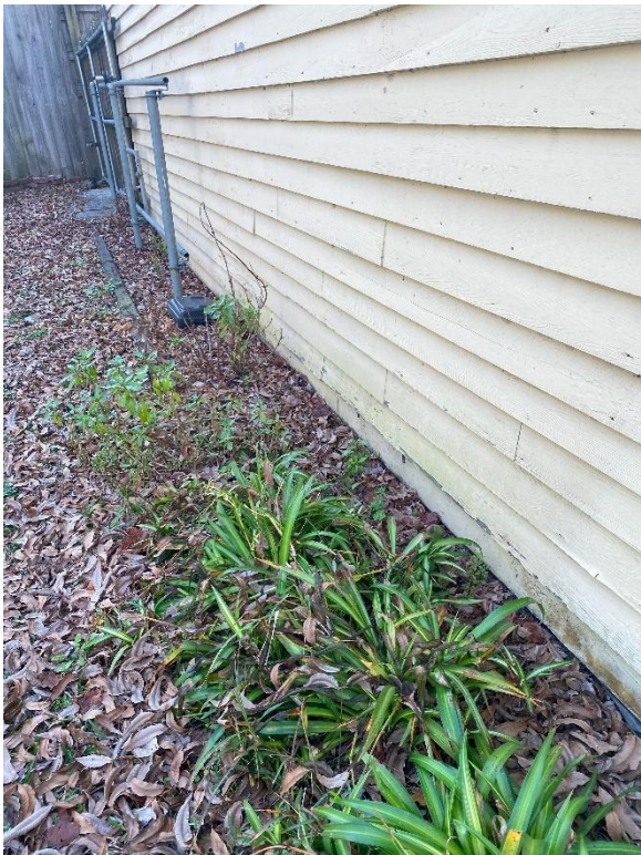
Lower boards below grade and other misc. damage
