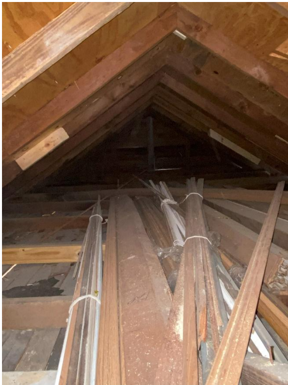
New rafters and roof sheathing
