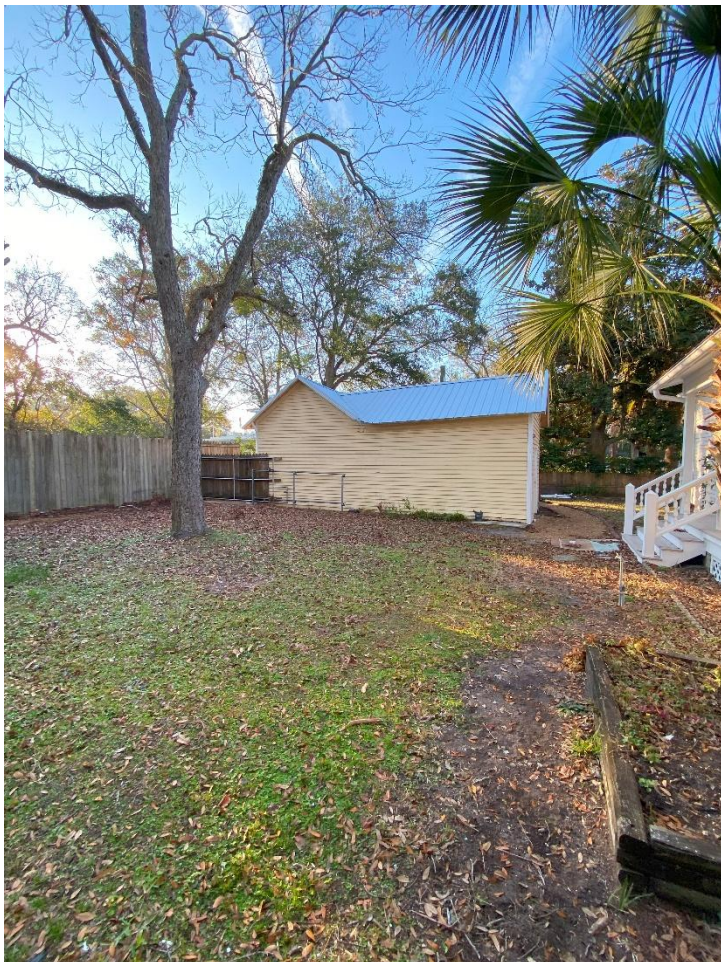
General overview of garage
