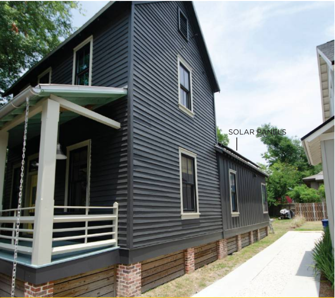
SOLAR PANEL PLACEMENT 322 North 3rd Street
