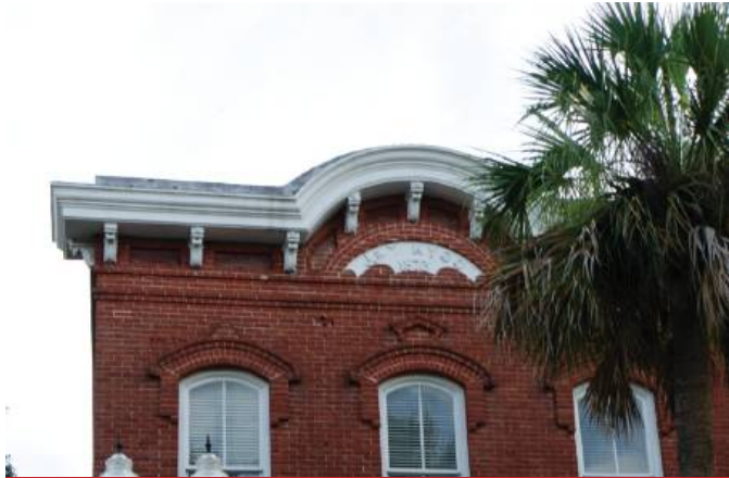
DECORATIVE BRICK CORBELLING 301 Centre Street
