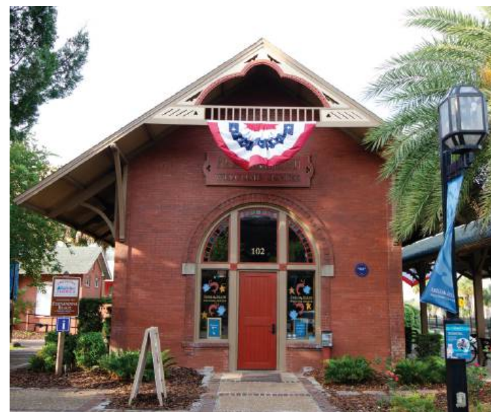
BRICK EXTERIOR 102 Centre Street
