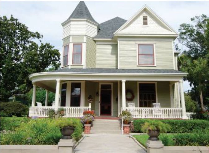
CONTRASTING PAINT COLORS 117 North 6th Street
