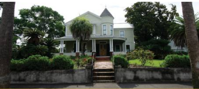
CONCRETE RETAINING WALL 112 North 6th Street
