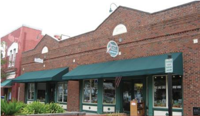
INFILL COMMERCIAL BUILDING 105-107 Centre Street
