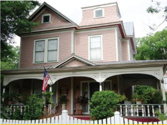
DECORATIVE BRACKETS 215 South 7th Street
