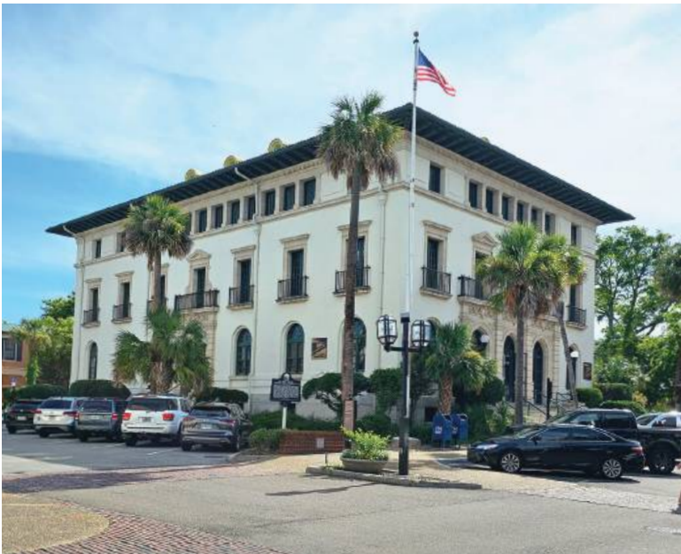
Post Office and Customs House, 401 Centre Street, 1912: Completed in 1912, the Post Office and Custom House is a beautiful example of Italian Renaissance Revival architecture. The architect was John Know Taylor, a relative of the 12th President of the United States, Zachary Taylor.
