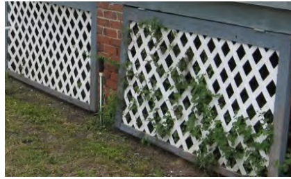
Wood lattices are appropriately fit into openings between brick piers of the foundation (910 San Fernando Street, above and 212 Estrada Street, below).
