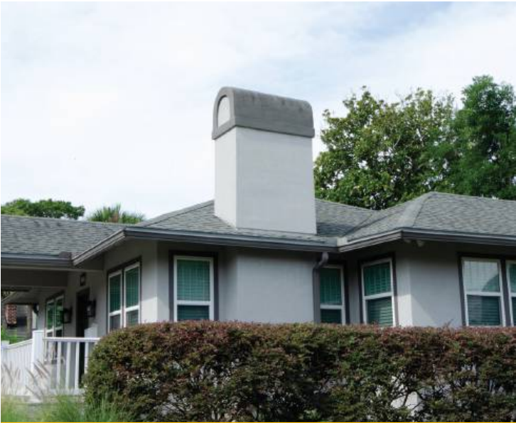
ROUNDED CHIMNEY 129 North 4th Street
