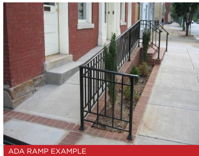
ADA RAMP 14 South Second Street
