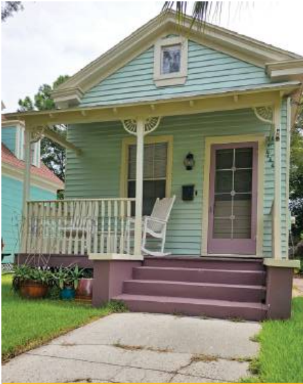
PORCH STAIRS & RAILING 414 South 7th Street
