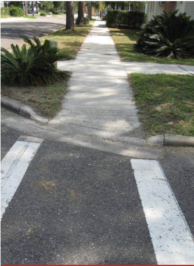
ADA CURBING South 7th Street
