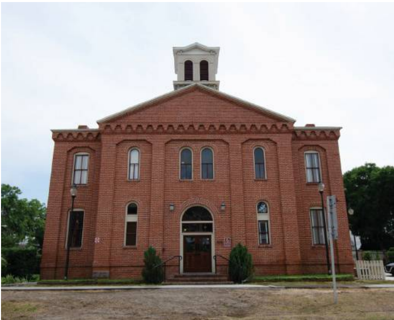
Amelia Schoolhouse Inn, 914 Centre Street, 1886: This robust brick Romanesque Revival school building was another example of the work of Master Architect Robert S. Skylar. It served as a school until 1927. It was adapted for use as offices in the 1980s and is presently a bed and breakfast inn.
