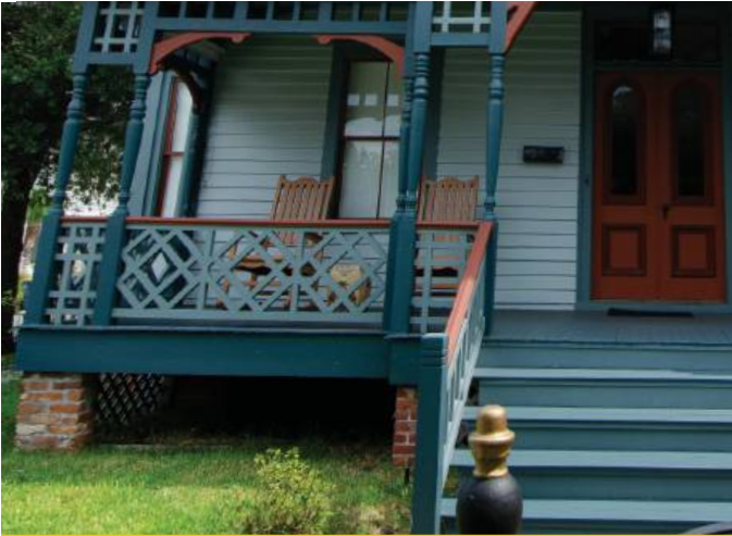
VISIBLE FOUNDATIONS 601 Ash Street
