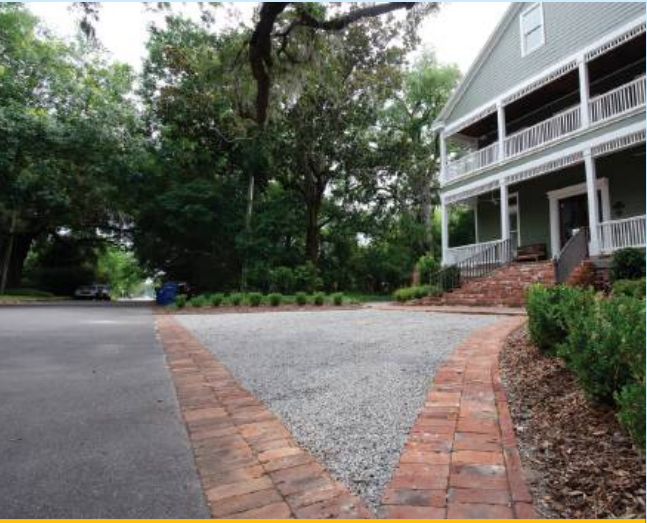
HISTORICAL PERVIOUS SURFACE 103 South 10th St.
