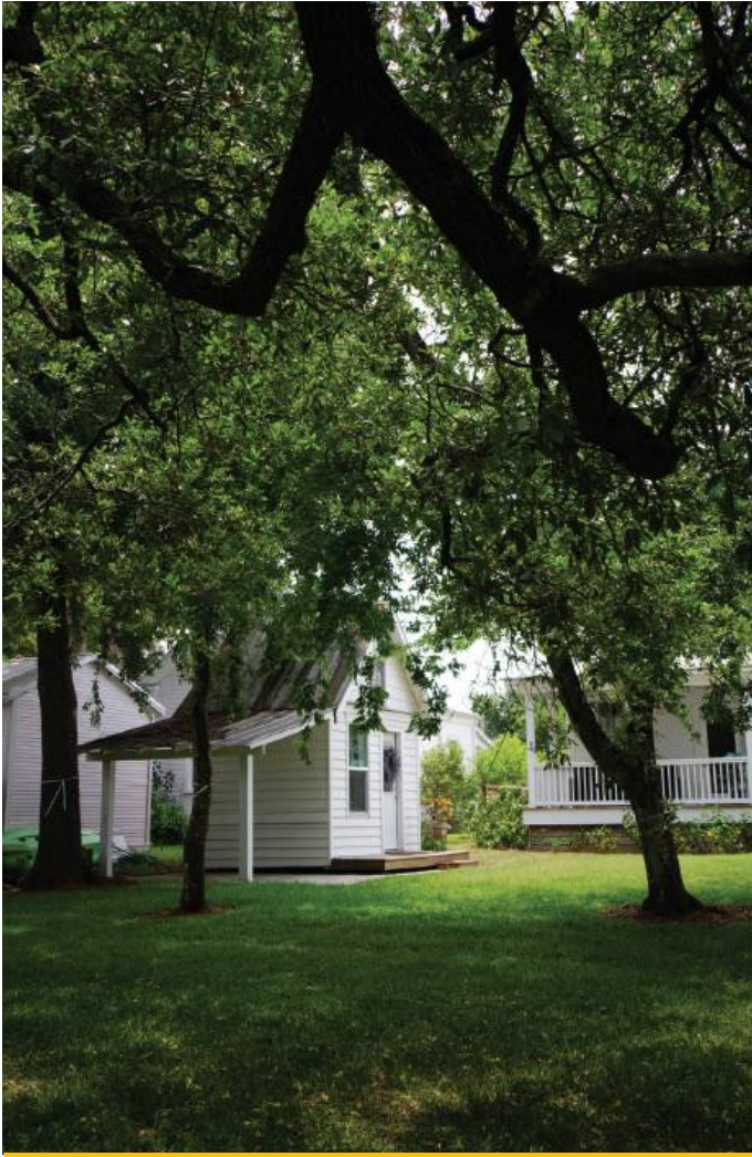
OUTBUILDING SHED 416 North 3rd Street
