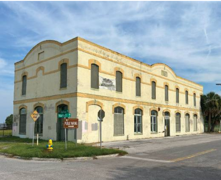
Huot's 1882 Building, 101-107 N. 2nd Street, 1882: This second building of C.H. Huot of France also housed his lumber and merchandise businesses. For most of the 20th century it housed Standard Marine Supply Company, a well-known business serving Fernandina's shipping and shrimping industry.
