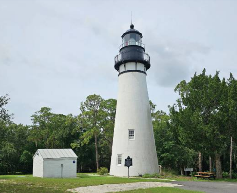
The Amelia Island Lighthouse, 215 O Hagan Ln, 1838: Built in 1838, the lighthouse has been an island landmark for over 150 years. The lighthouse has been upgraded several times and continues to be operated by the U.S. Coast Guard. The building is open for tours on a periodic basis.
