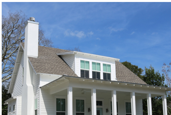
Gable with Dormer Window
