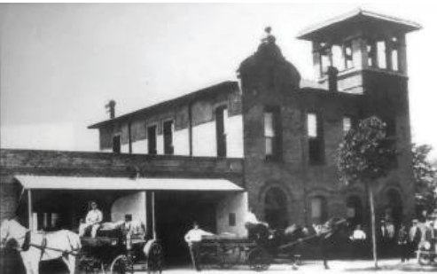
CITY HALL STRUCTURE IN 1915
