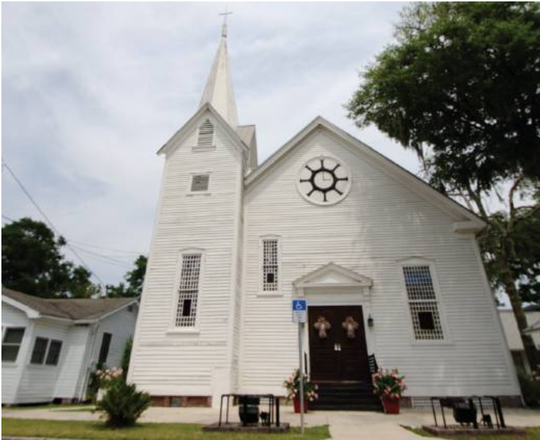
First Missionary Baptist Church, 1874: This Carpenter Gothic Church was completed in 1874 for Fernandina's African American community. It features a bell tower, steeple and a circular spoked window on its main façade.
