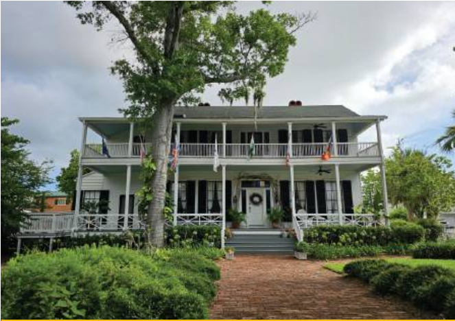
BRICK WALKWAY 415 Centre Street
