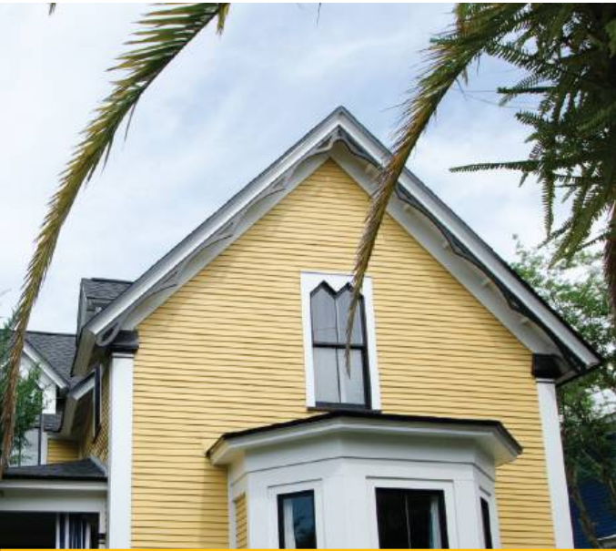
2X2 WINDOW 17 South 7th Street
