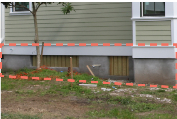
Figure 30: Examples of the types of foundations encouraged in the District. Foundations include brick, stone, lattice, stucco, and horizontal or vertical boards.
