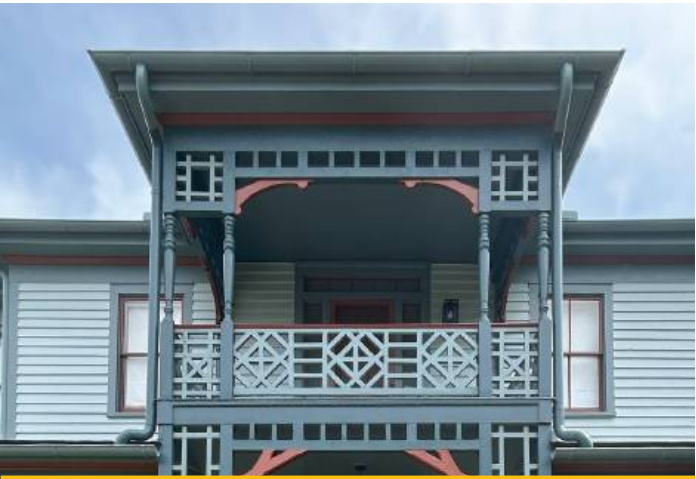
DECORATIVE TRIM 601 Ash Street
