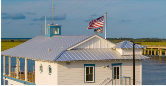
Roofing-aluminum standing seam -silver finish
