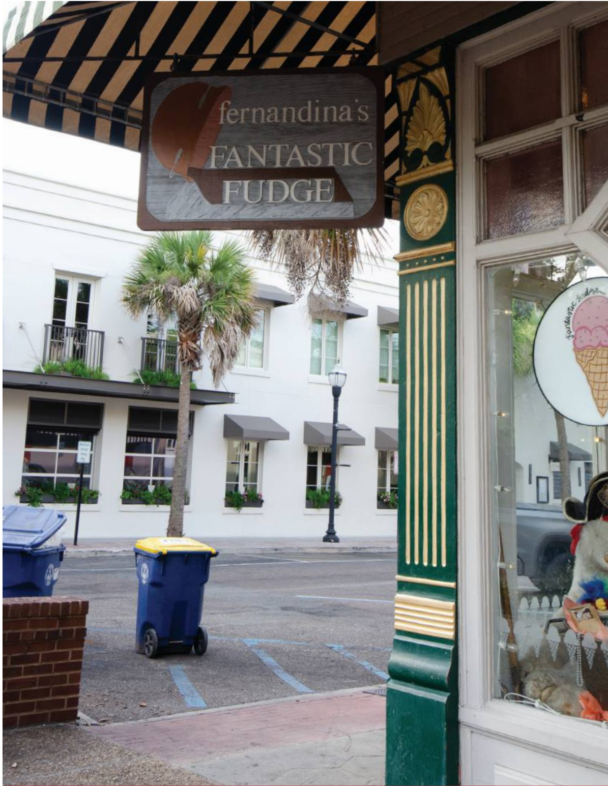
PAINTED METAL SURFACE 218 Centre Street
