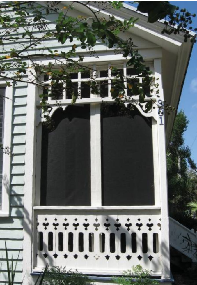
SCREENED PORCH 301 South 6th Street
