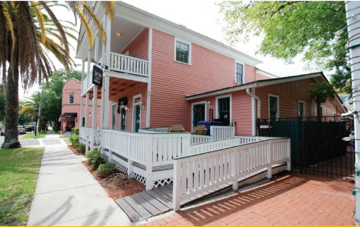
ACCESSIBILITY RAMP 218 Ash Street
