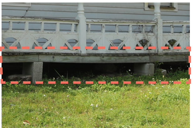
Figure 30: Examples of the types of foundations encouraged in the District. Foundations include brick, stone, lattice, stucco, and horizontal or vertical boards.
