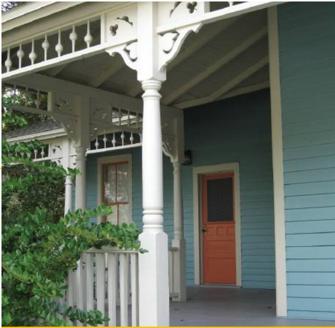
PORCH FEATURES 28 North 4th Street
