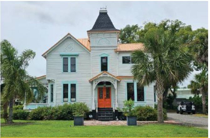
PAINTED EXTERIOR & TRIM 303 South 8th Street
