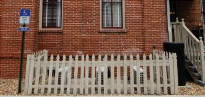
FENCED UTILITIES PLACEMENT EXAMPLE
