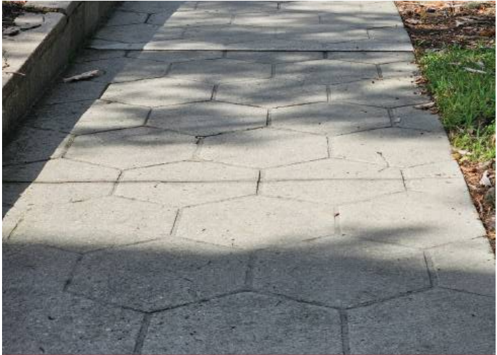
HEXAGON BLOCK WALKWAY 2 North 6th Street
