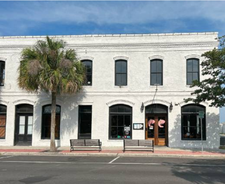
Seydel Building, 29-31 N 2nd Street, 1877: Constructed in 1877, this handsome brick building housed the millinery and general store of A. Seydel and Brother, German immigrants.
