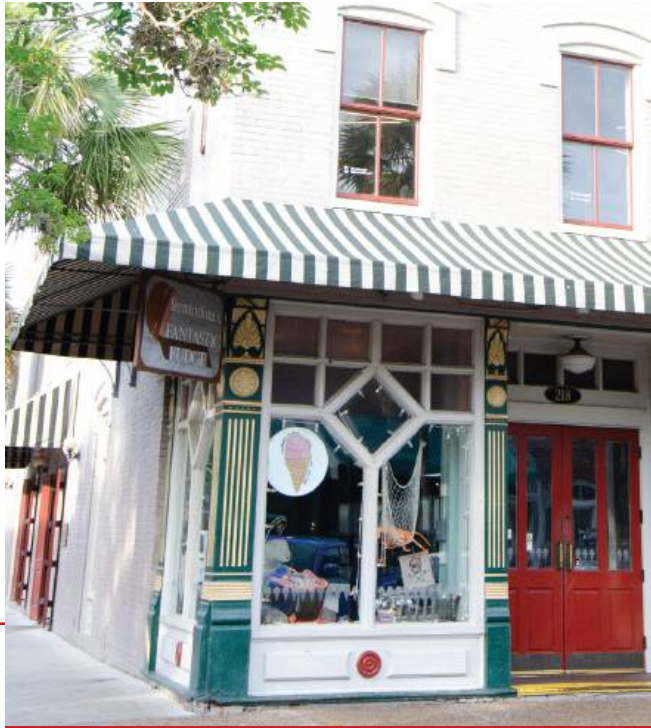
STOREFRONT BULKHEADS 218 Centre Street
