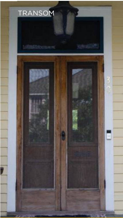
ENTRANCE 319 South 3rd Street
