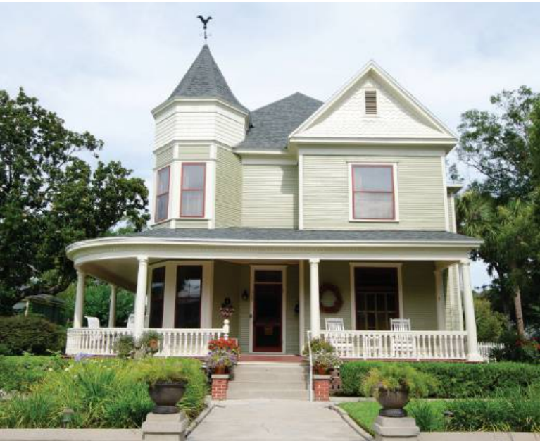
Humphreys House, 117 N. 6th Street, c. 1900: Built c. 1900 by master builder George Watts, who also built the strikingly similar Horsey House, the Humphreys’s House is an outstanding local example of the Queen Anne style. The original owner was Dr. D.G. Humphrey who shared a practice with Dr. H.J. Horsey.
