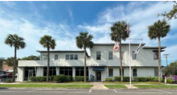
CITY HALL STRUCTURE NOW
