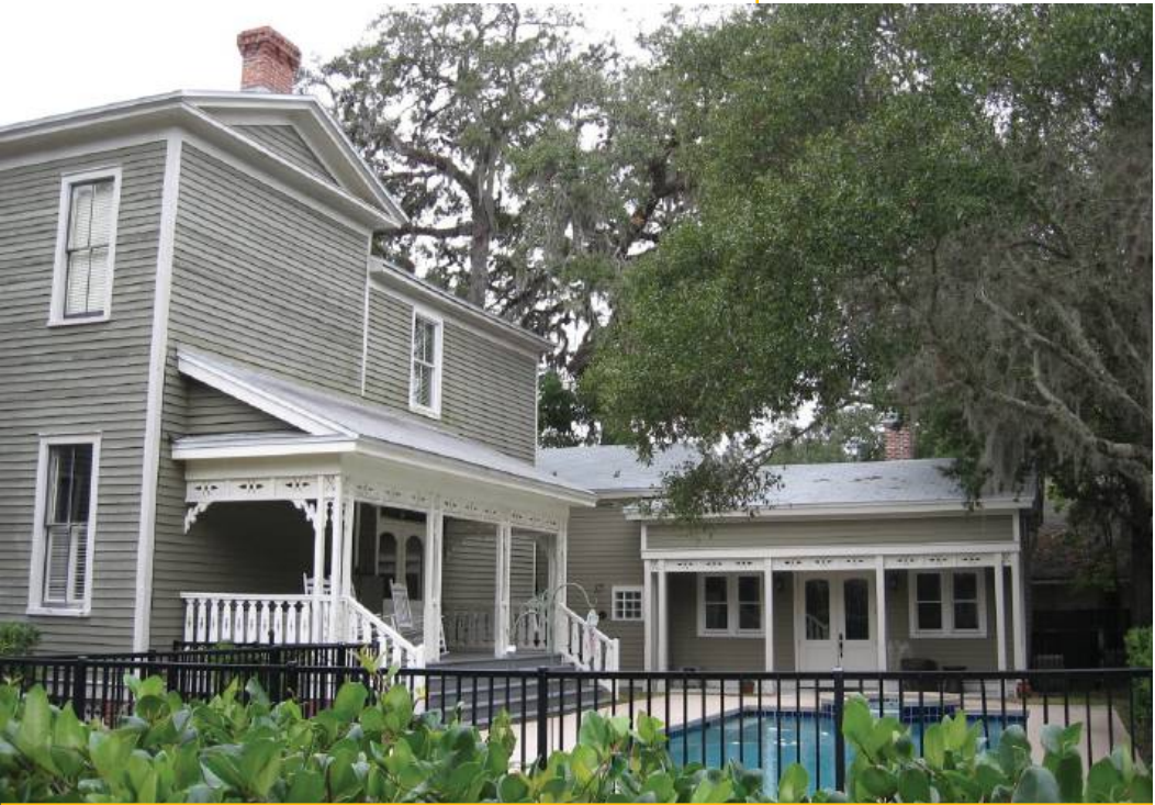
LATERAL WING ADDITION 31 South 10th Street
