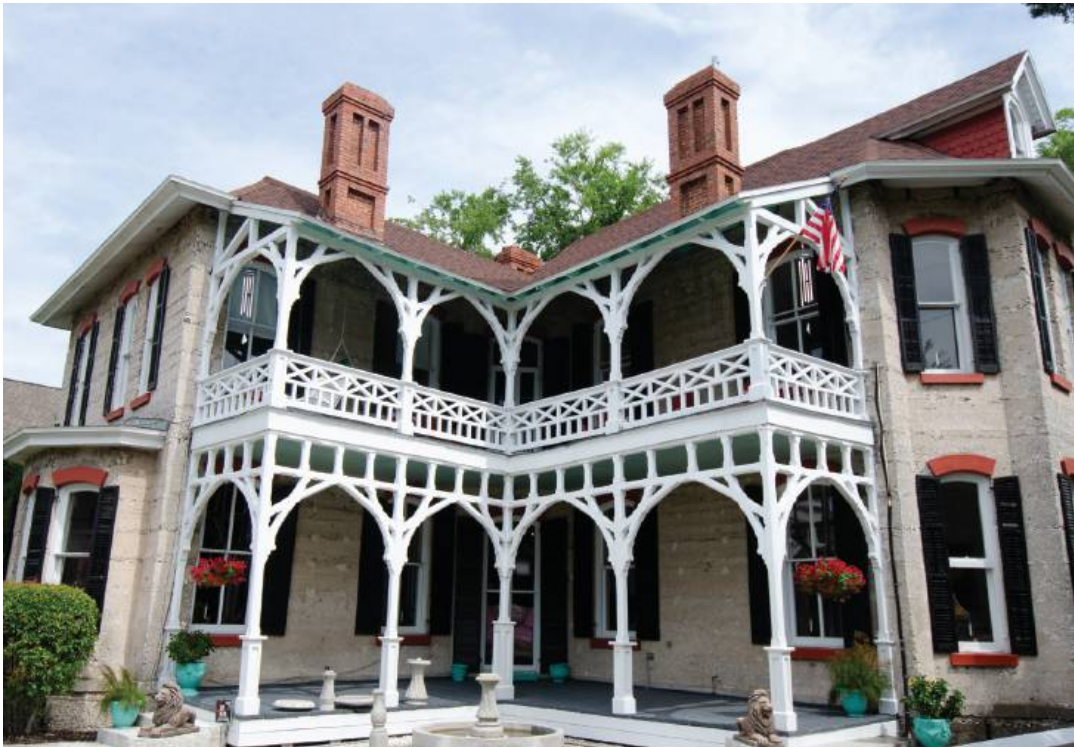
JIGSAW PORCH RAILING DESIGN 27 South 7th Street
