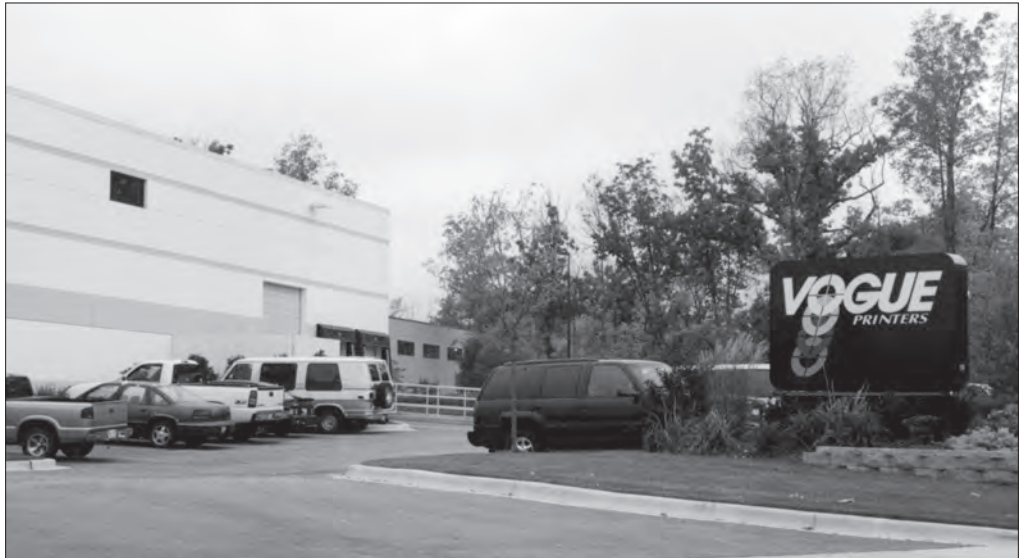
printing and publishing facility
