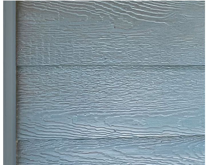
Figure 14. Surface texture is an important aspect in matching the appearance of a historic material, especially when a material is viewed at close range. As seen in these two images, many of the substitute materials produced for siding and trim have an embossed wood grain, making them incompatible for replacing historic wood that was typically planed to a smooth surface. Some substitute products are available with a smooth surface as well. Photos: John Sandor, NPS.
