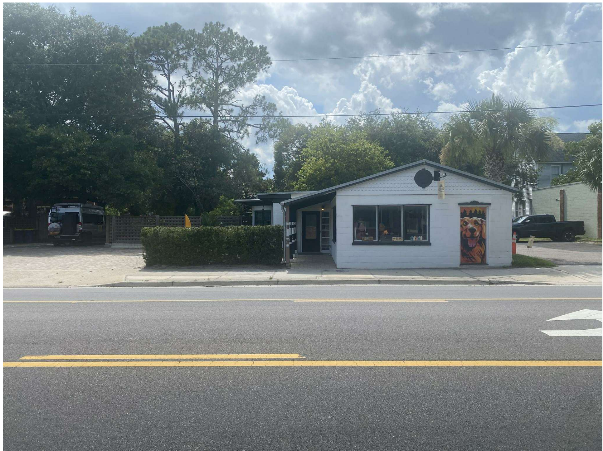
EAST ELEVATION STREET VIEW
