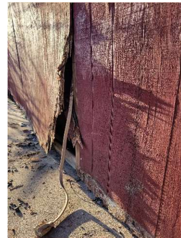
Exterior North Wall, East Bottom Area Exterior Covering
