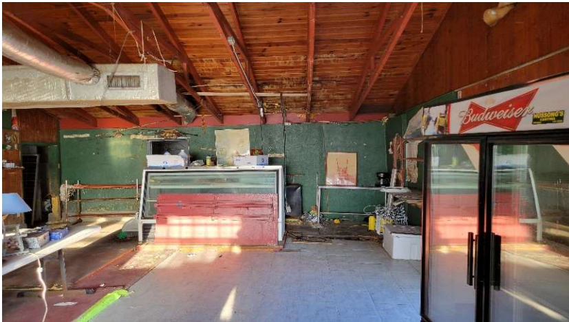
Main Room – Looking West
