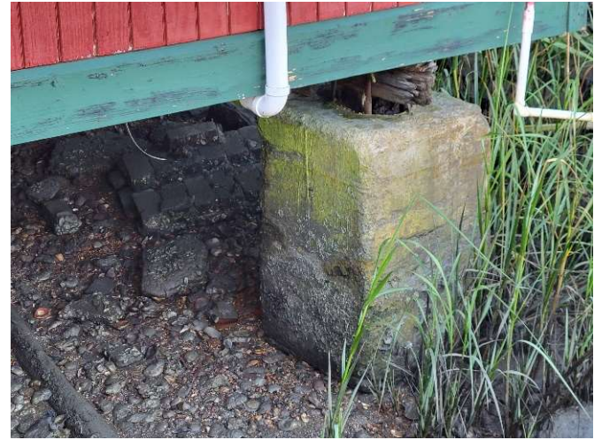
Exterior Southwest Column & Girder
