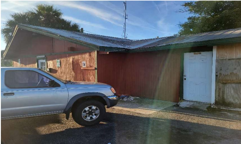
North Exterior Wall
