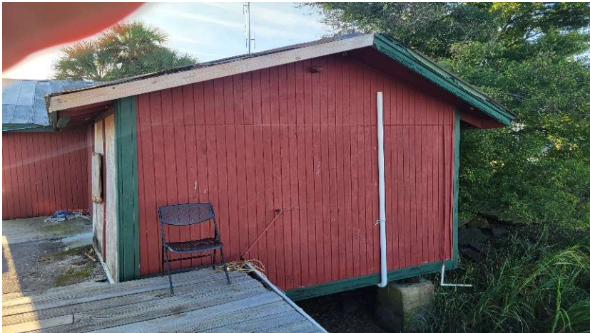
West Exterior Wall
