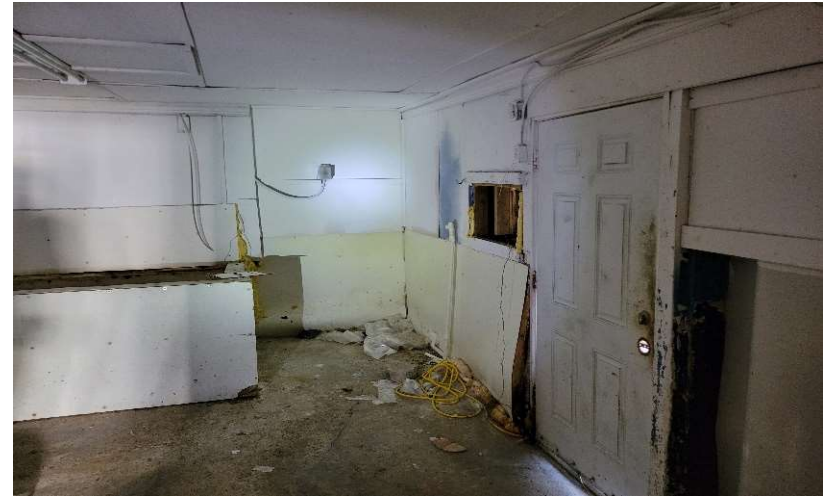
Fish Room – Looking Northwest
