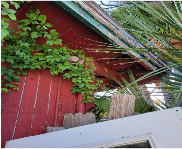
Exterior Eave Southeast Corner
