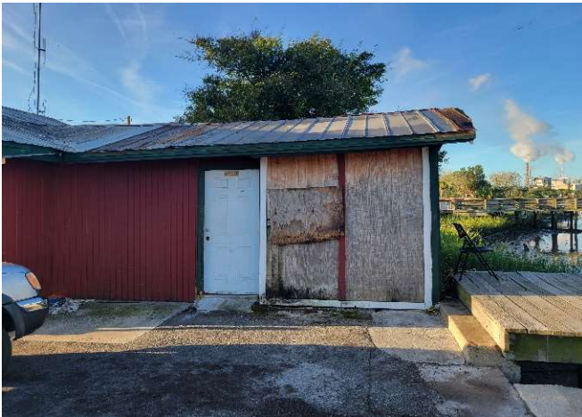
Exterior North Wall, West Addition
