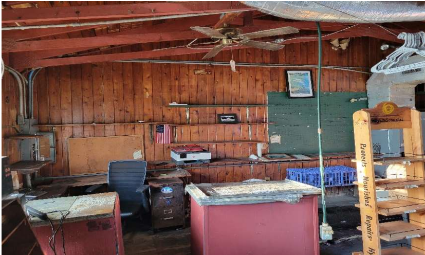
Main Room – Looking South
