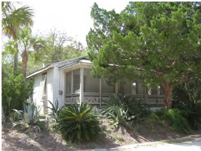
The mid-20th century dwelling at 1012 Ladies Street is non-contributing but rehabilitation work should respect its original design and detailing.
