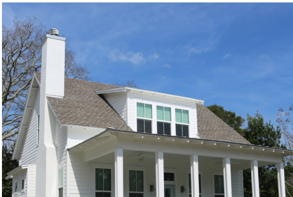
Gable with Dormer Window
