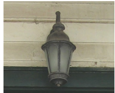
Retain original light fixtures or those added in the early 20th century (212 Estrada Street).
