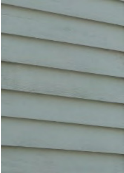
Original wood siding at 808 San Fernando Street.
