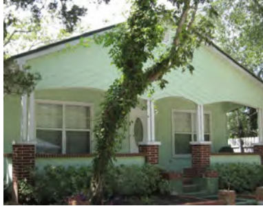
A wide porch with posts on brick piers is a character-defining feature of this Bungalow dwelling (906 Someruelos Street).
