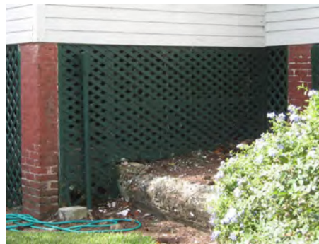
Wood lattices are appropriately fit into openings between brick piers of the foundation (910 San Fernando Street, above and 212 Estrada Street, below).
