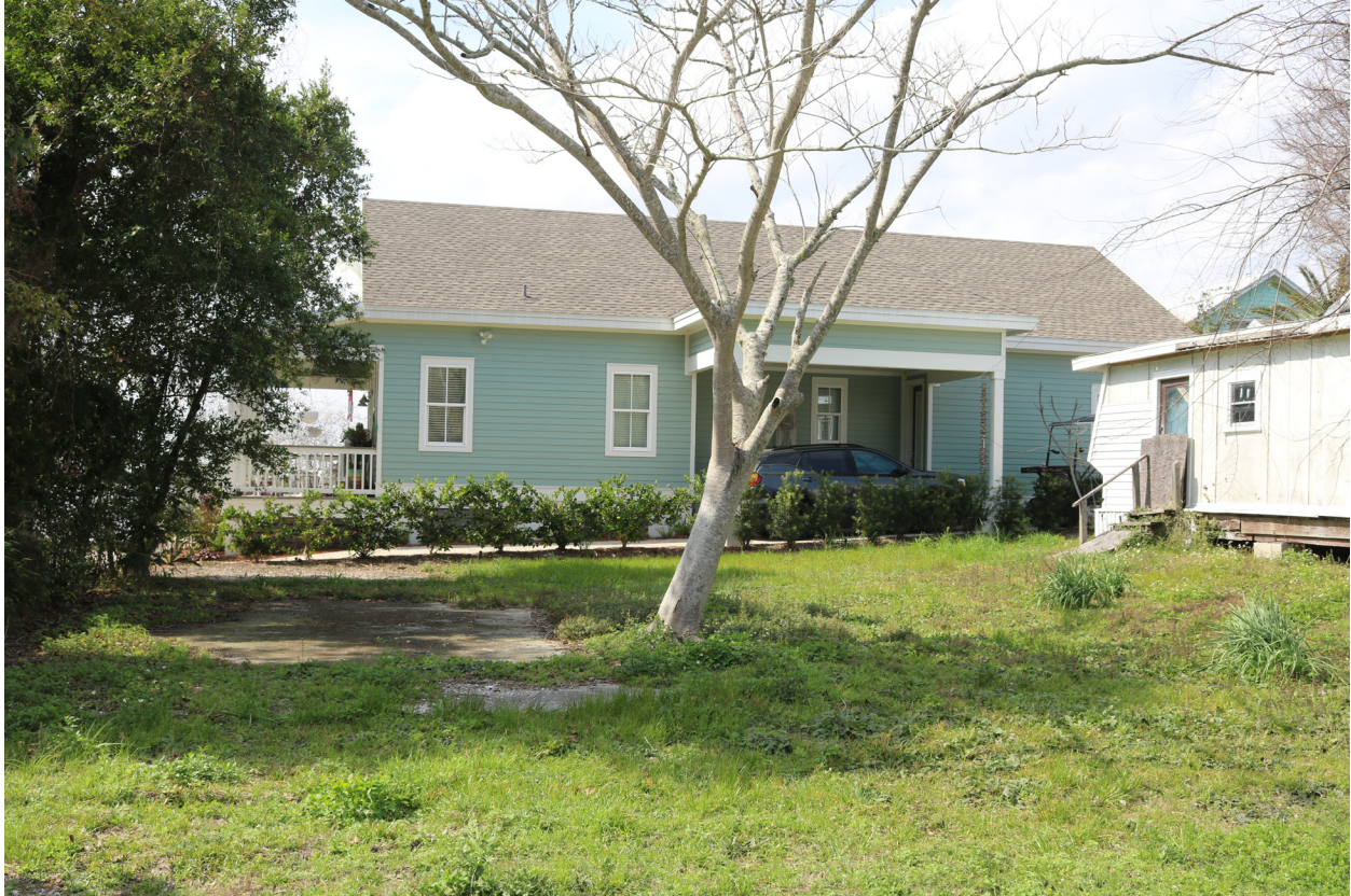
Carports are allowed, but limited in size to accommodate two cars maximum.
