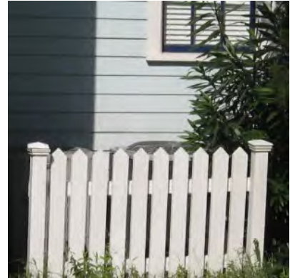
Appropriate screening of HVAC unit (715 San Fernando Street).
