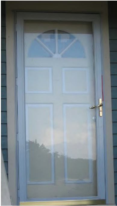
This appropriate storm door allows for view of the door behind it (117 Estrada Street).
