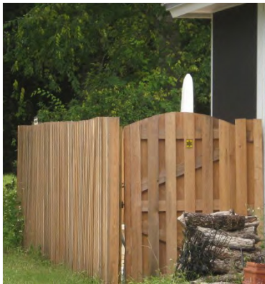
This privacy fence is an appropriate location and design in the back yard of 902 San Fernando Street.
