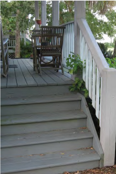
These porch steps are appropriate designs for rebuilding stairs on older houses or for new construction (115 Estrada Street).
