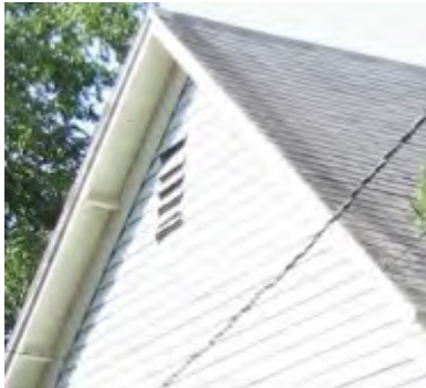
Original roof shapes should be retained (808 San Fernando Street).
