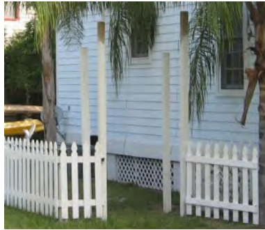
Appropriate wood picket fence design at 807 White Street.
